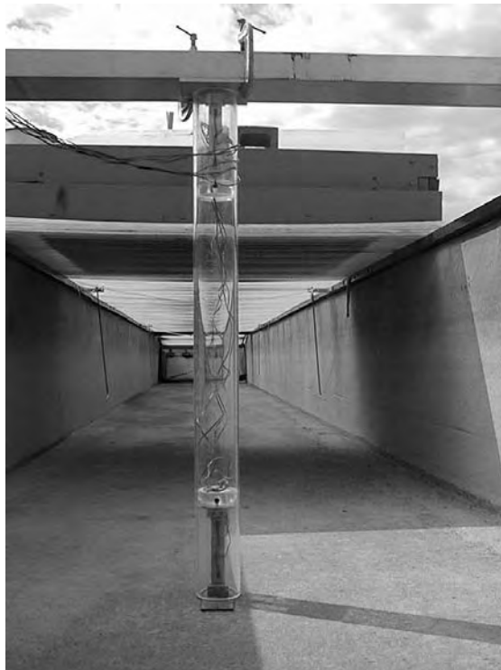
Figure 3.17: Pier installed in the channel
