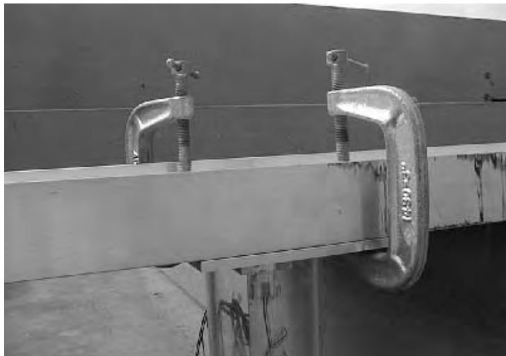
Figure 3.23: Fixing device for the top
