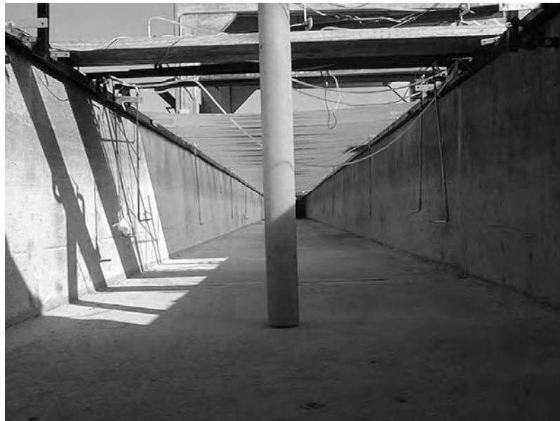
Figure 5.7: The 3.5 in. (8.9 cm) diameter roughened pipe in the middle of the channel's cross section
