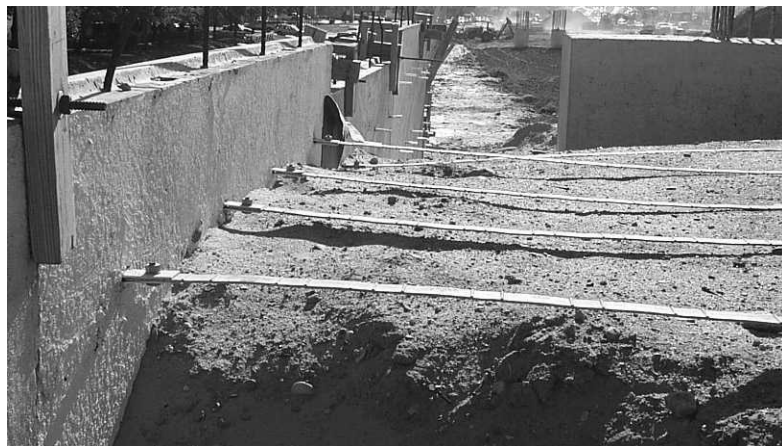
Figure 1.4 Typical ribbed steel strip reinforcement from MSE wall construction at IH-35 and US290 in Austin
