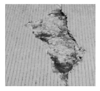
Figure 2.3 Example of deep delamination spalling
