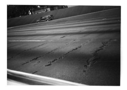
Figure E1 Typical spalling of a pavement
