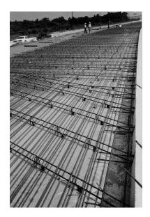
Figure 1.12 Metallic crack inducer located on top of longitudinal rebar
