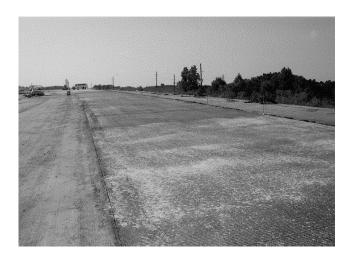
Figure 3.30 Linseed oil and water-based curing compound curing experiment
