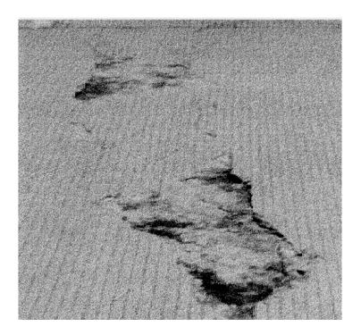
Figure 5.1 Typical example of spalling
