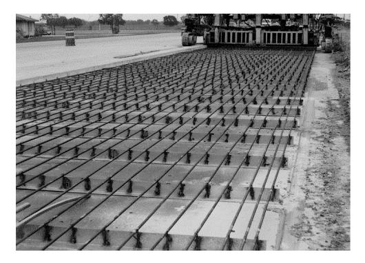
Figure 1.8 Type III crack inducer located in TS3
