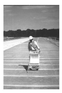
Figure 3.12 Longitudinal sawcutting using the early-entry method
