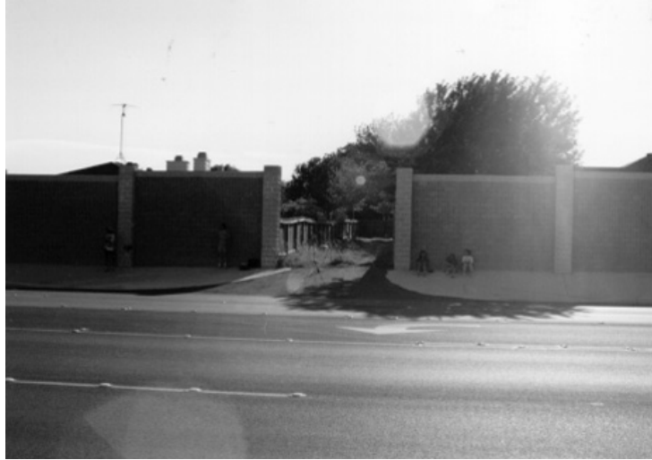
(a) Noise barrier opening at entrance of alley
