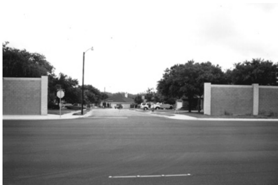
(a) Noise barrier opening at entrance
