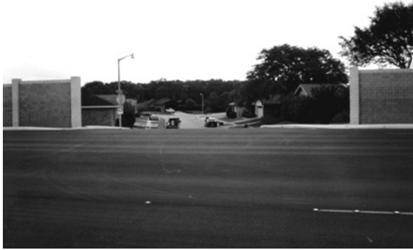
(a) Noise barrier opening at entrance (note elevation ref FM 3009)
