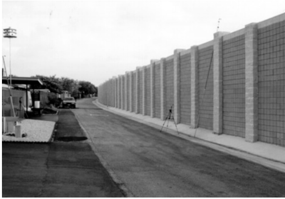
(a) Garage access alley behind noise barrier
