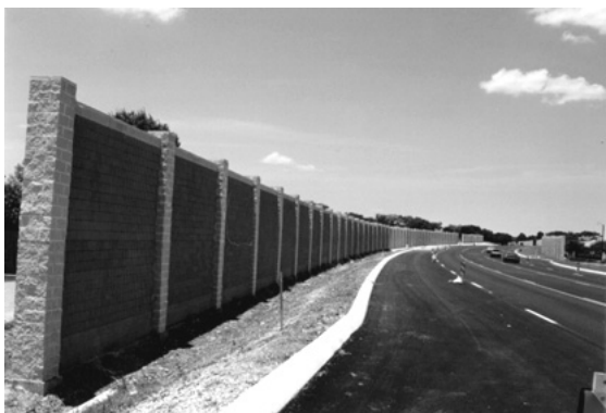
Figure 2.2(c) Barrier elevation difference at Eli Whitney
