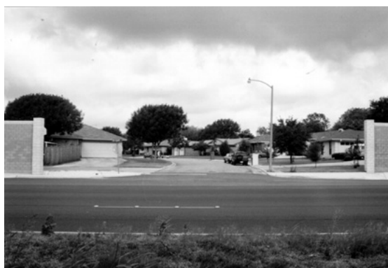
(a) Noise barrier opening at entrance
