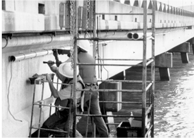
Figure 5.2: Conduit installation
