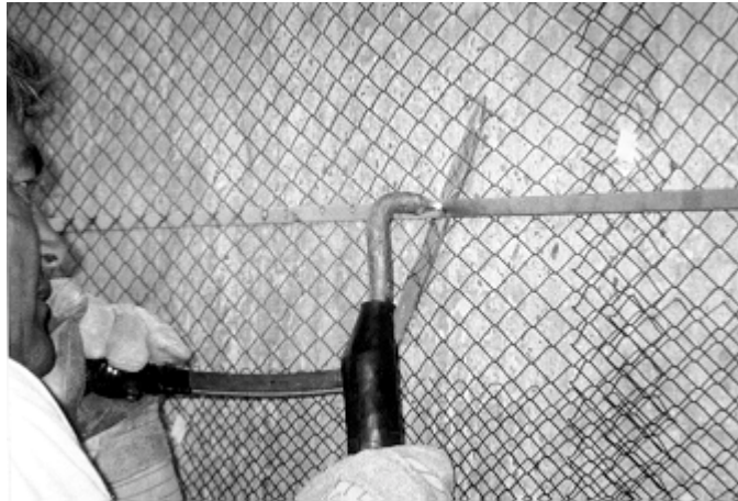
Figure 5.13: Spot welding of titanium strip to titanium mesh
