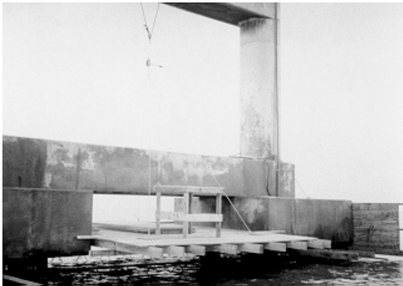
Figure 5.1: Modified scaffold design in raised position
