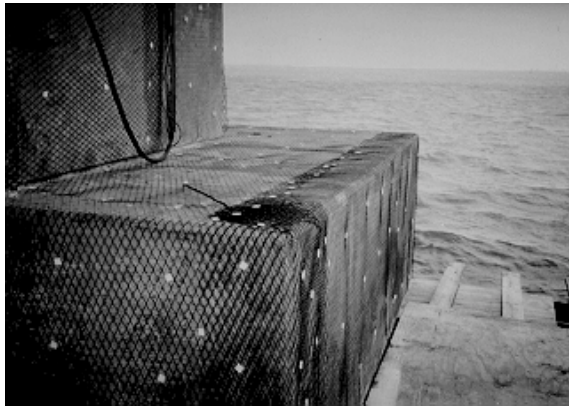
Figure 5.12: Titanium mesh secured with plastic fasteners
