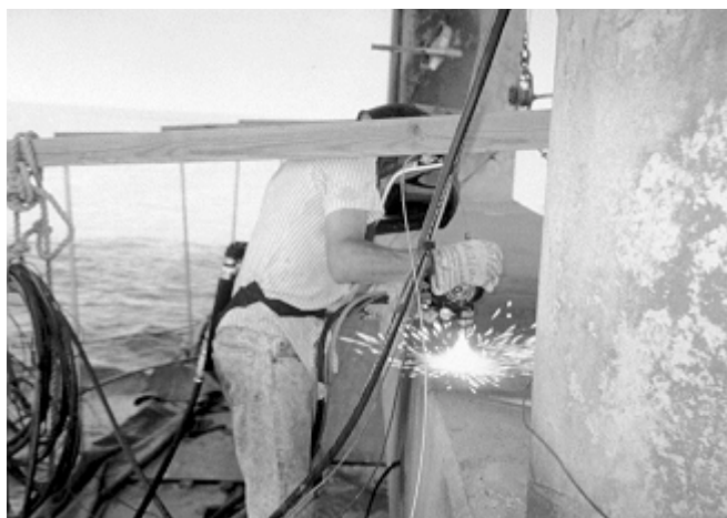
Figure 5.11: Titanium flame spraying
