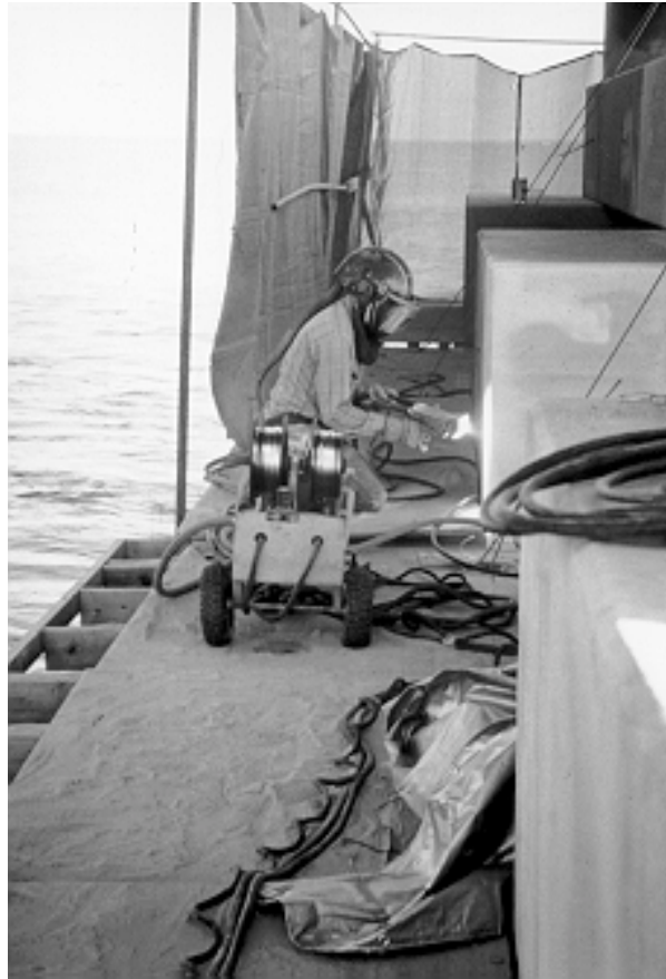
Figure 5.8: Zinc arc spraying
