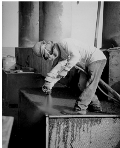
Figure 5.15: Shotcrete application of titanium overlay
