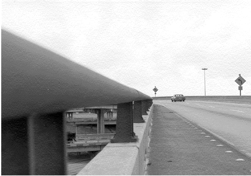
Photo 2.7 Warning Signs and Flashers Before and On the Curve
