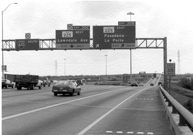
Photo 2.6 Gore of Exit Ramp
