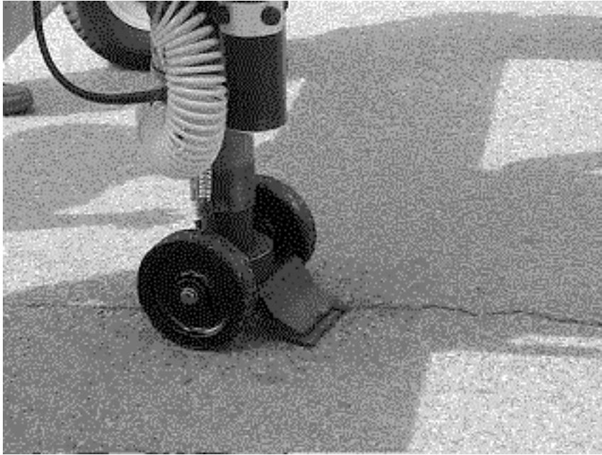
Figure 5.10. The ARMM Sealing Cracks without the Sealant Material
