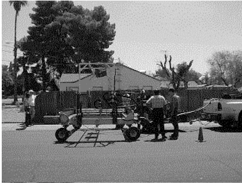
Figure 5.29. The Demo Location close to Crafcro Headquarters
