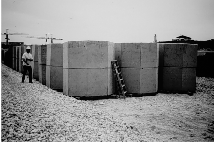
Figure 1.6 - Precast Bridge Pier Segments
