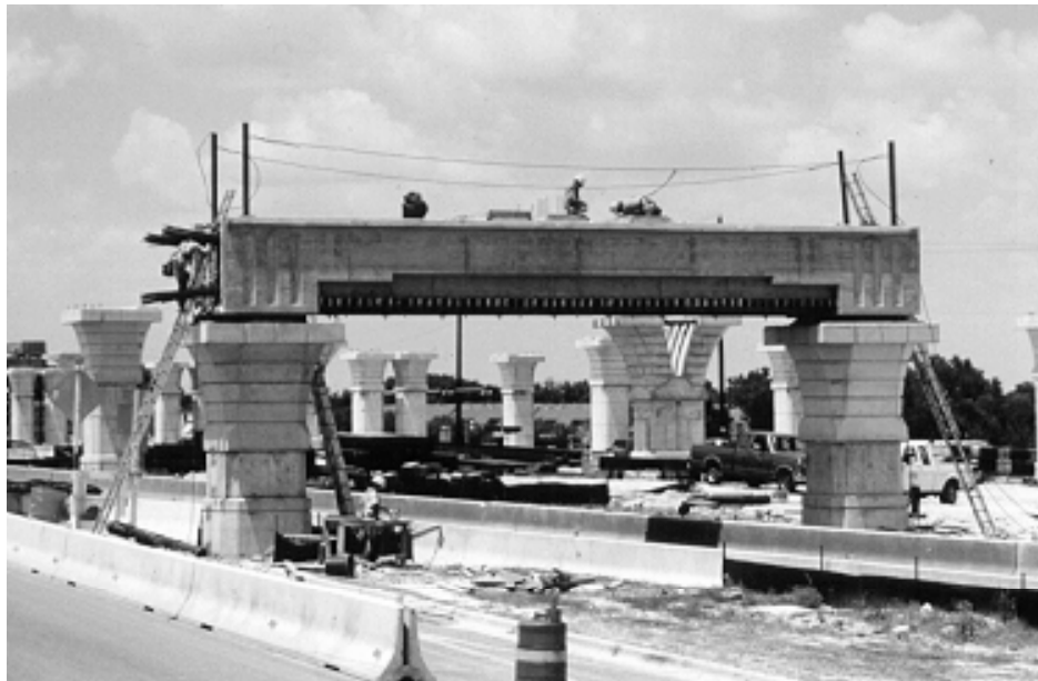
Figure 1.7 - Post-Tensioned Straddle Bent
