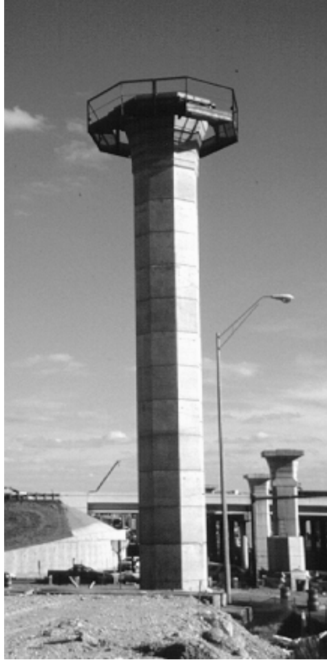
Figure 1.4 - Post-Tensioned Precast Segmental Bridge Pier
