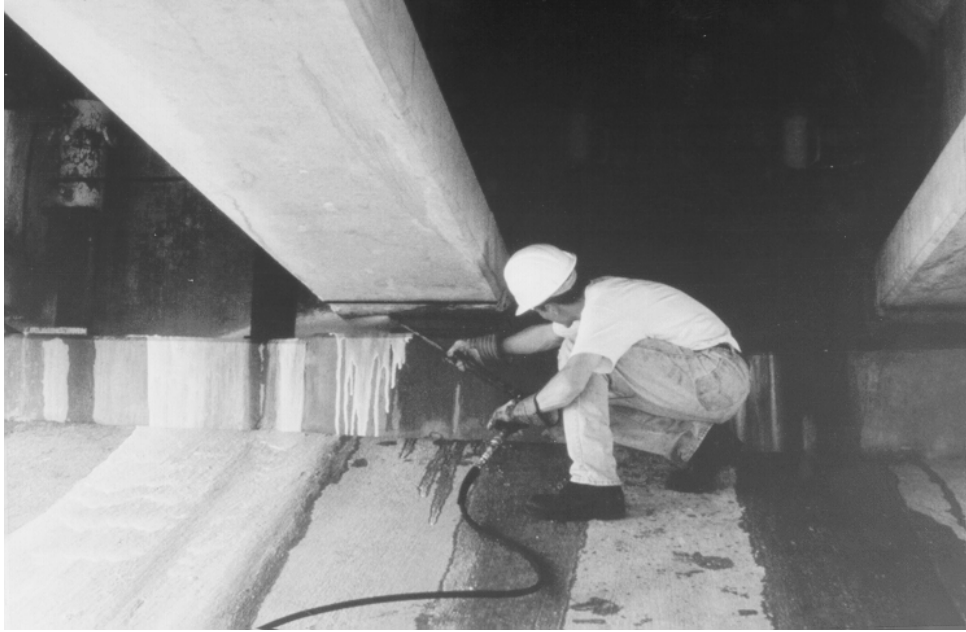
Figure 3- 13 Steam cleaning the girders and bearing seats with degreasing agent
