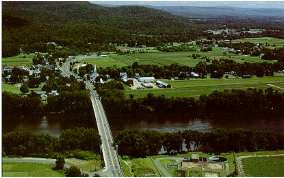
Figure 15. Rte. 116 Bridge (D06003) in Deerfield, MA
