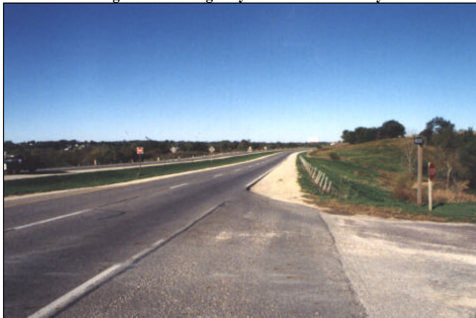
Figure 63: US Highway 69 in Warren County
