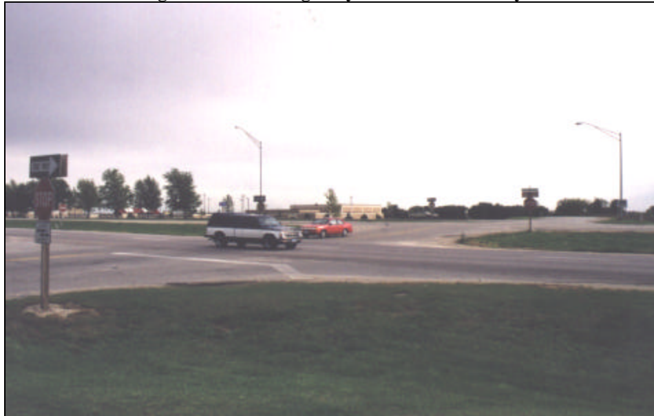
Figure 61: Iowa Highway 163 in Polk County
