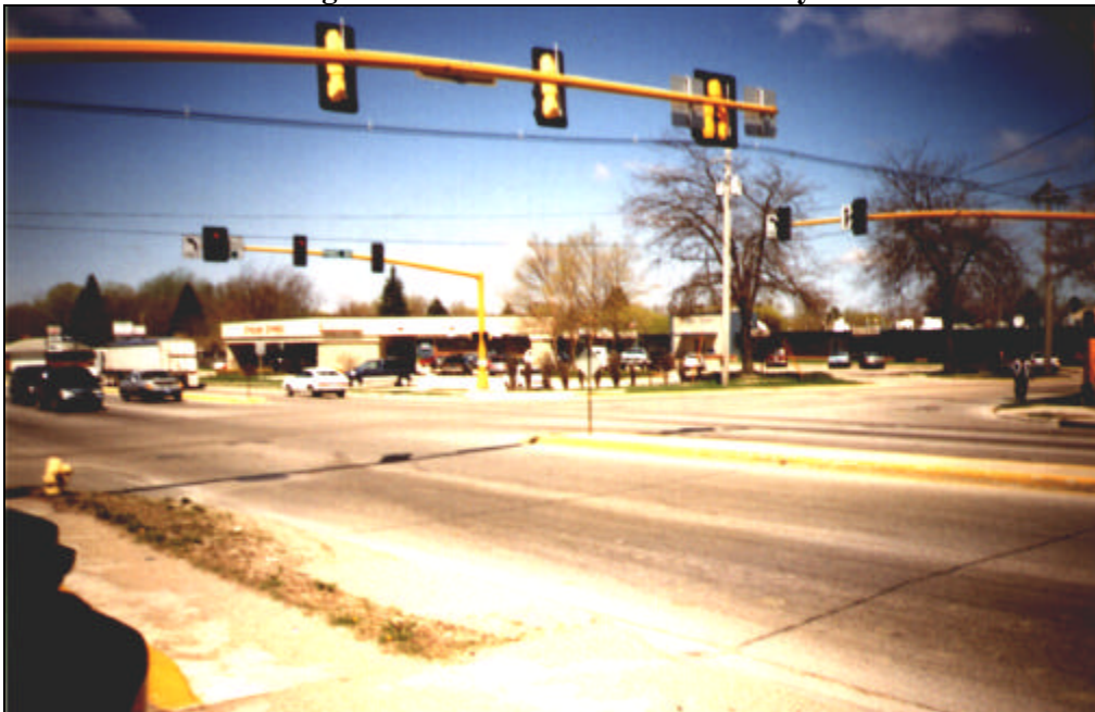
Figure 39: 4th Street Southwest Today
