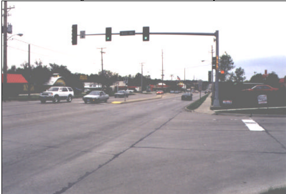
Figure 28: Northwest 86th Street Today
