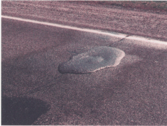
1 Deposit sufficient slurry to fill crack.
