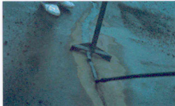
3 Strike off sealant with squeegee to create overband.
