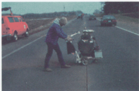
1 Rout cracks.
