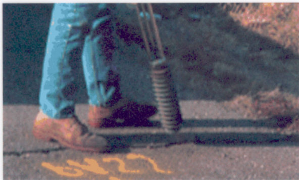
1 Dry thoroughly with hot-air lance or high-pressure air hose.
