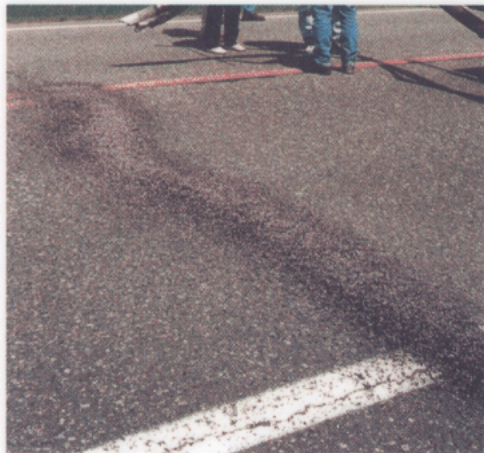
1 Spray injection crack repair
