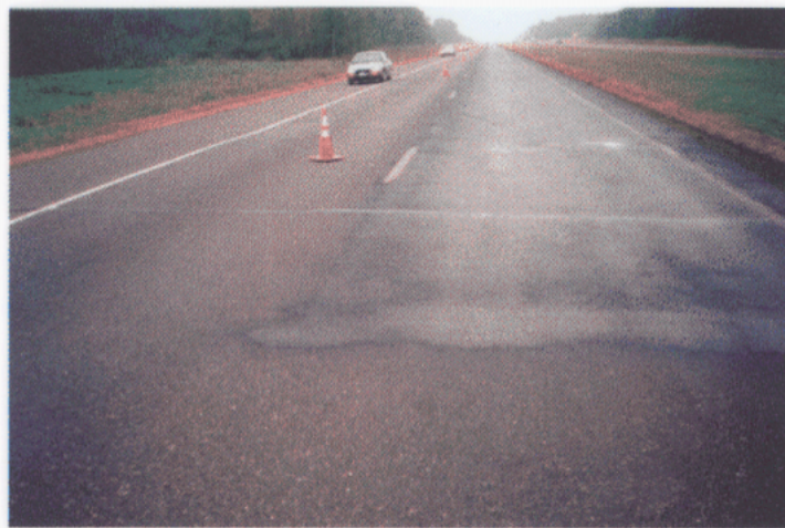
Pavement should be dry and clean before fog sealing.
