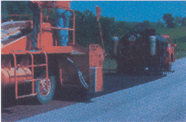
1 Minimize the distance between the binder distributor and aggregate spreader.
