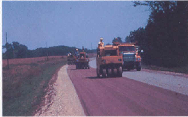
2 Use a minimum of three rollers, all at 5 mph maximum speed.
