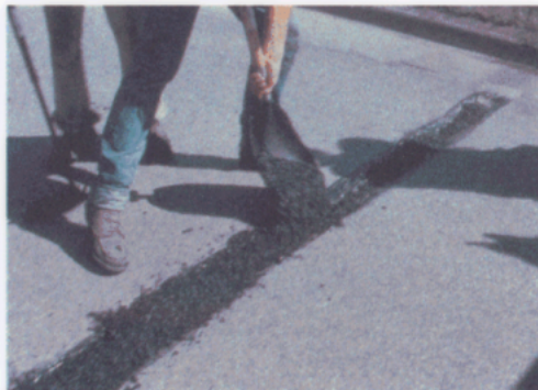
3 Place hot mix neatly in reservoir.
