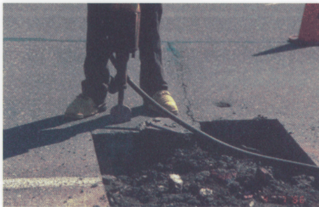
2 Remove as much pavement as needed to reach firm support.
