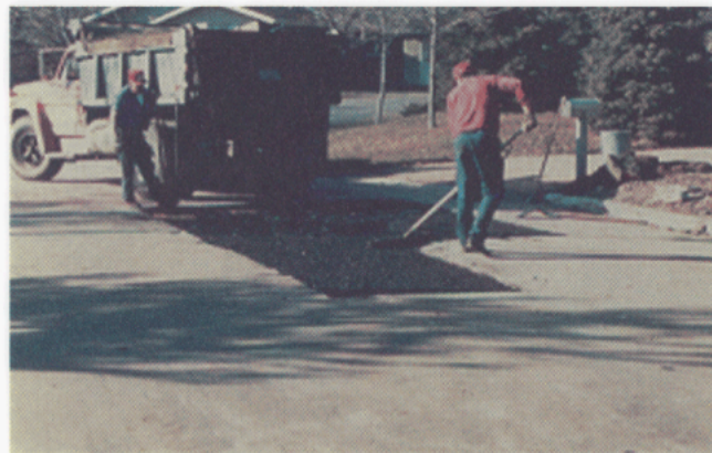
3 Place patching material in hole and compact.
