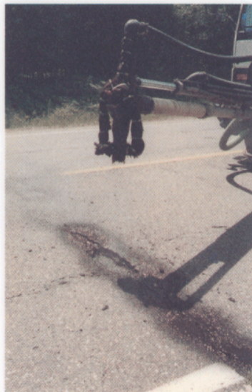
2 Spray injection patching used on a pothole
