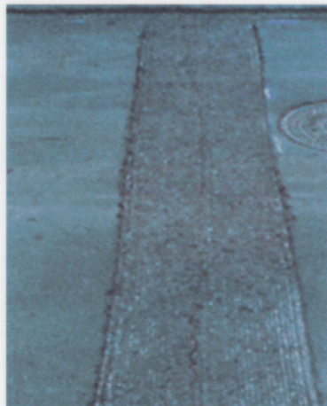
2 A clean reservoir ready for new hot mix
