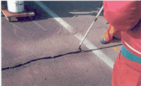
2 Fill clean crack with sealant.
