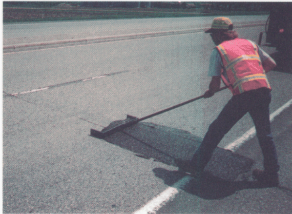
2 Strike off slurry material.
