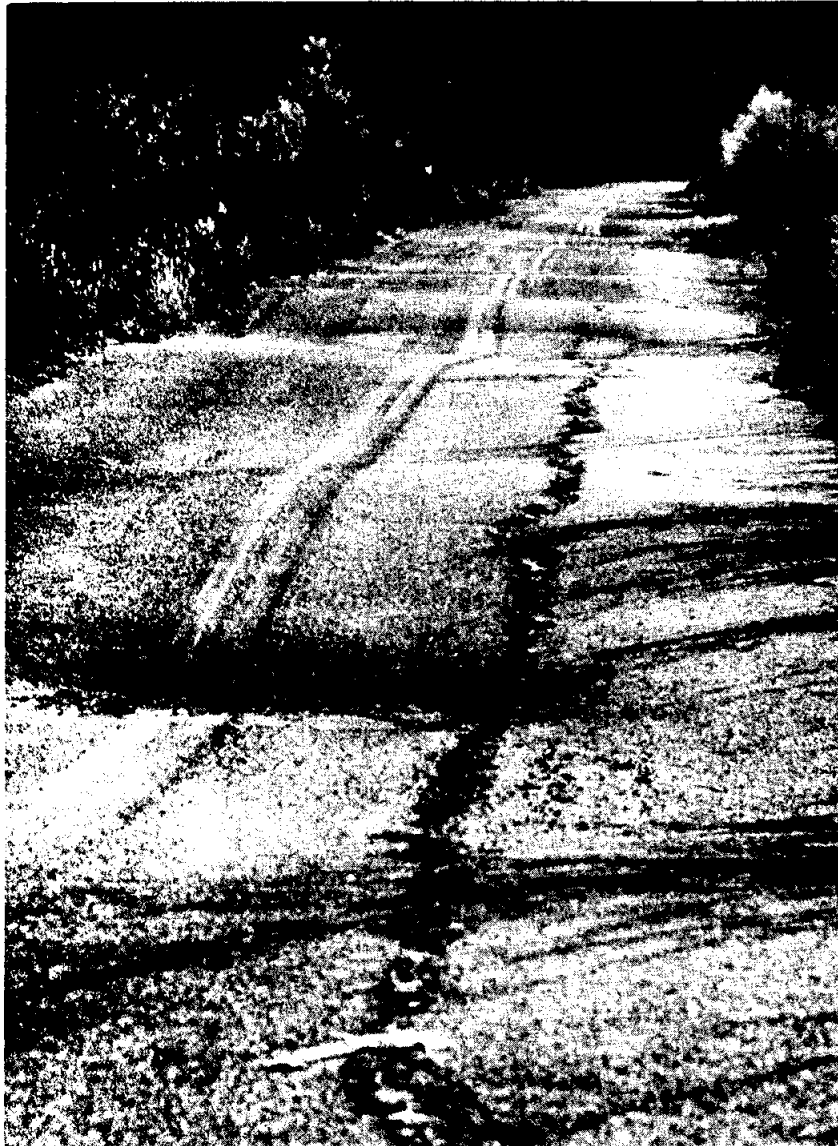
Photo 2. Road roughness resulting from thaw settlement
