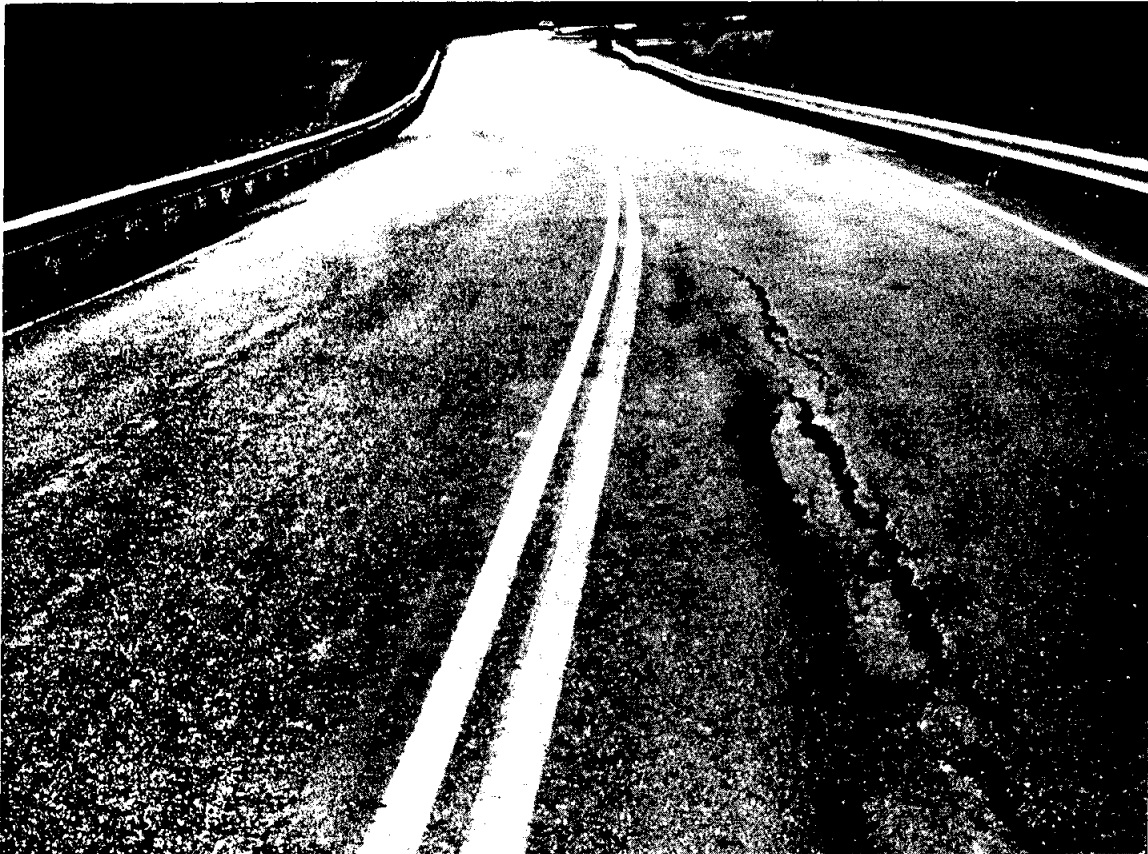
Photo 6. A five layer section on Chena Hot Springs Road starts even with the wheel lying against the right guardrail. Longitudinal cracking and patching end at about this point, but settlement dips continue (note the sharp dip in the right guardrail).
