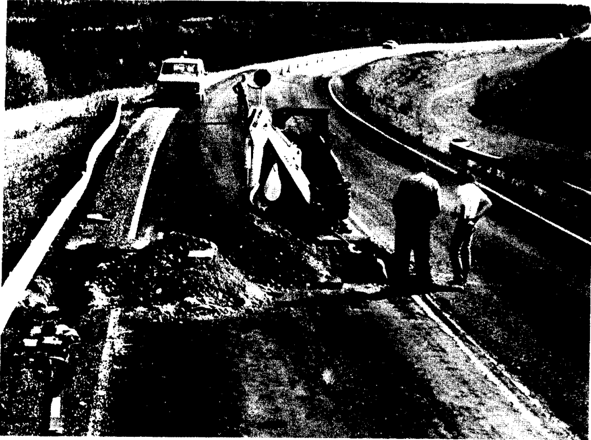
Photo 8. Excavation of 5 layer section on Chena Hot Springs Road, June, 1987.
