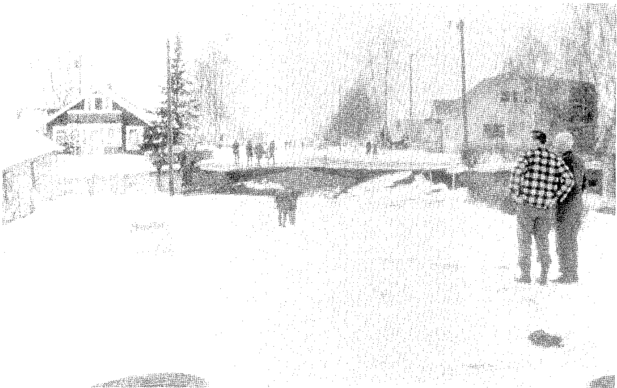
Figure 3(b) - L Street Slide Damage
