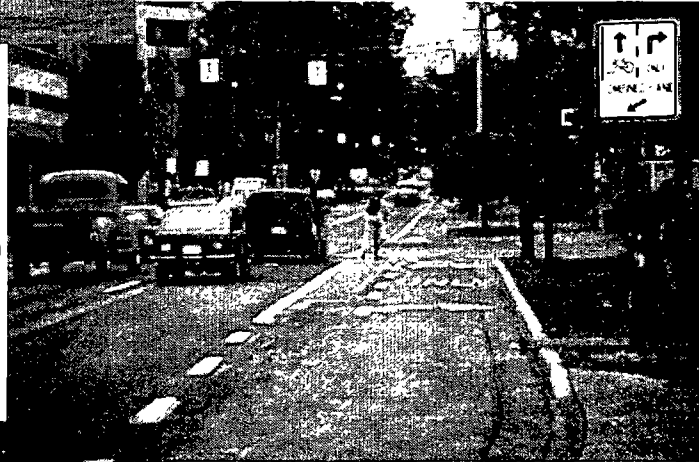
High-volume, low-speed intersection with unique combined right-turn/bicycle lane.
