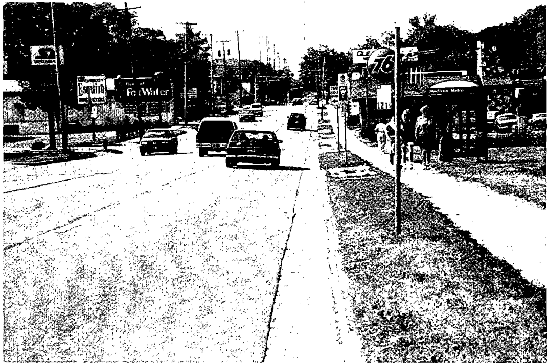
Figure 3. High-volume multilane pilot study site with an 85th percentile speed of 55 km/h and a curb lane width of 3.4 m.
