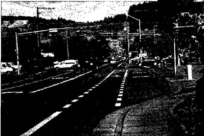
Low-volume, low-speed intersection with bicycle lane separated from motor-vehicle lanes by wide-dashed striping.
