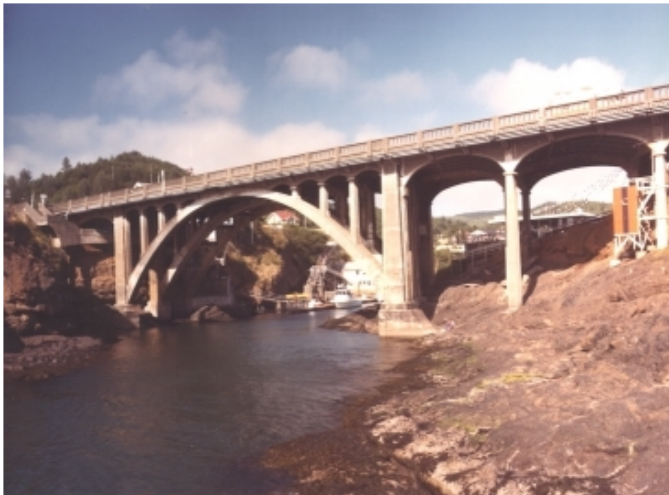
Figure 6.1: Depoe Bay Bridge
