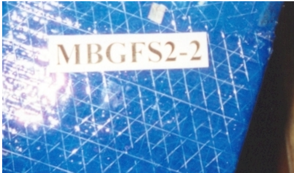
Figure 3.11: Typical appearance of MBrace™ GFRP system.
