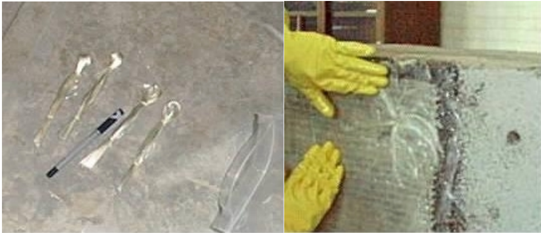
Figure 3.7: Typical Tyfo® system glass anchors (left), and typical appearance of applied anchor in concrete beam (right).
