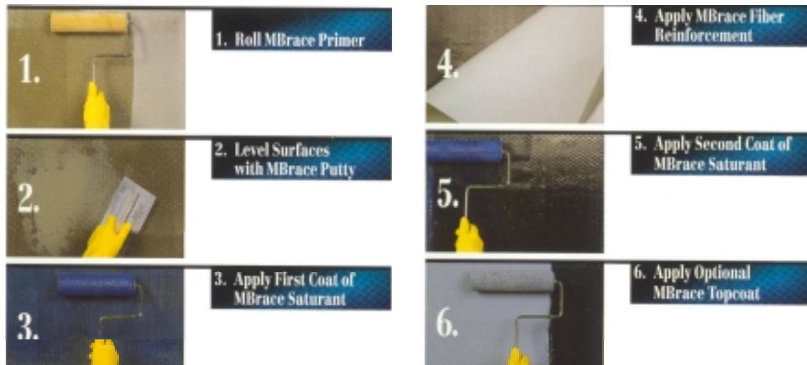
Figure 3.1: MBrace™ Application Procedure ( Master Builders, 1997 )
