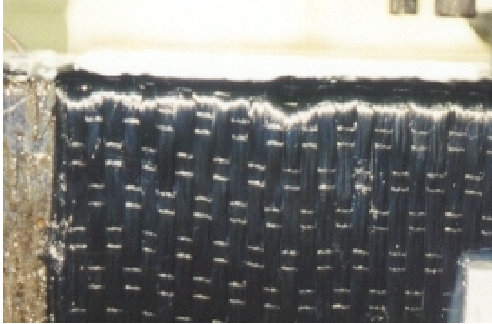
Figure 3.6: Typical appearance of SikaWrap® Hex FRP system.
