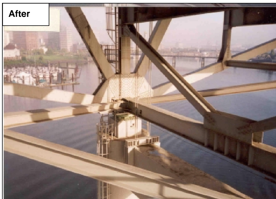
Figure 3.10B: New Bearings on Pier #4
