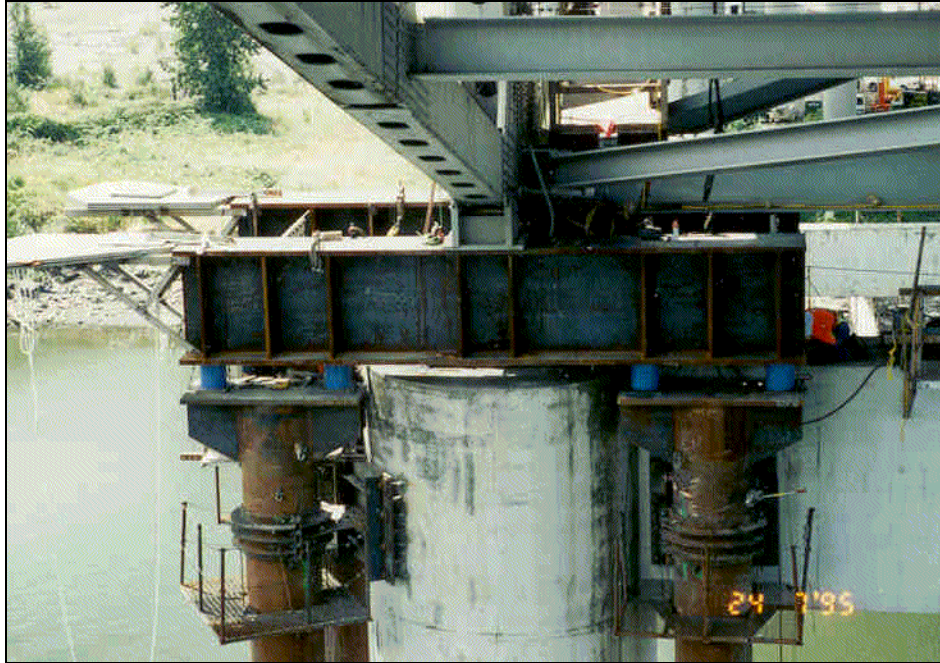
Figure 3.7: The Lifting Assembly for Piers #3 and #4
