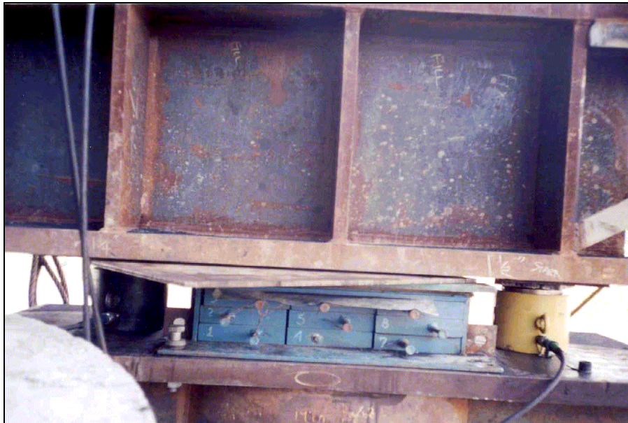
Figure 3.3: The Lifting Assembly for Piers #2 and #5
