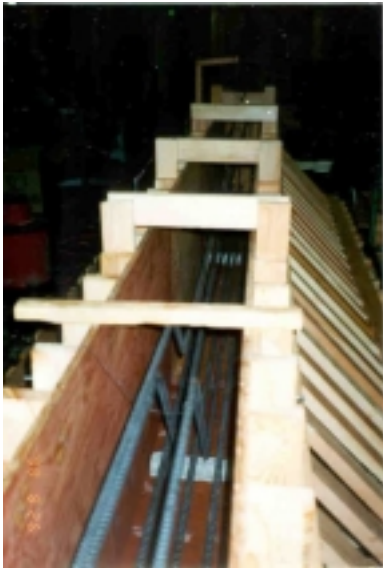
Figure A-4: Typical formwork w/ steel
