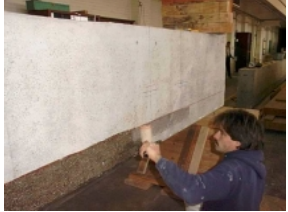
Figure A-10: Tack coat and epoxy application
