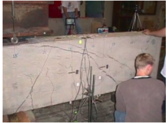
Figure A-23: Shear failure through sections
