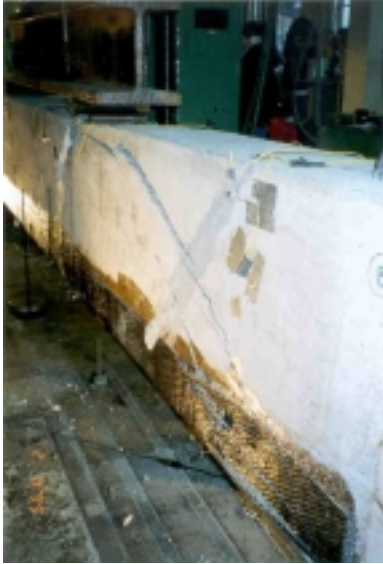
Figure A-31: Failure similar to Control beam
