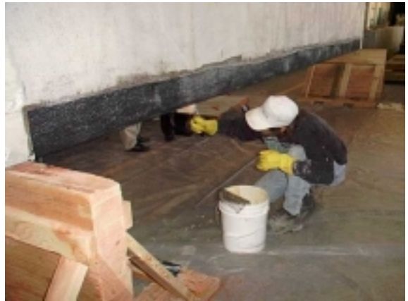
Figure A-17: Second coat of epoxy/CFRP
