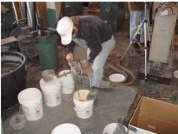
Figure A-15: In situ epoxy mixing
