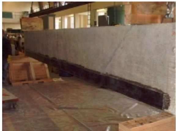
Figure A-18: Completed carbon reinforcement
