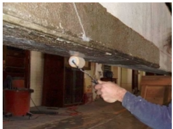
Figure A-12: Epoxy application
