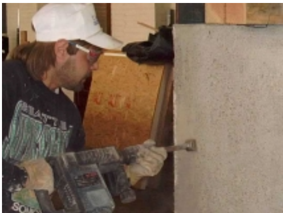
Figure A-8: Surface preparation: abrasion
