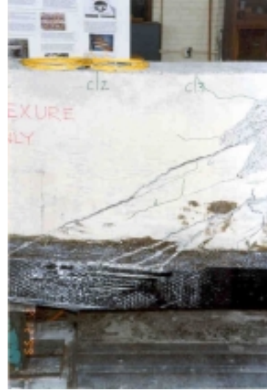
Figure A-34: Cracking at failure
