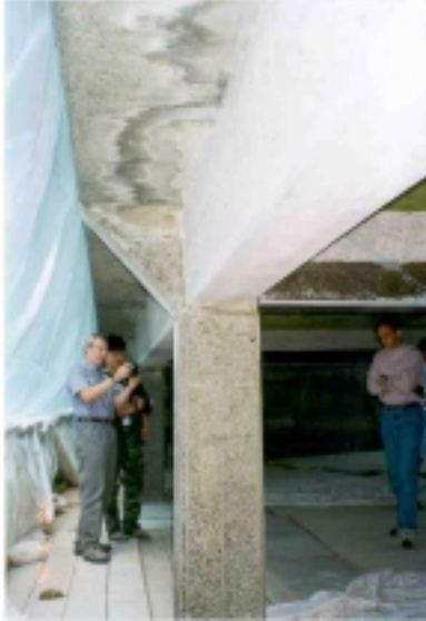
Figure A-3: Bridge during retrofit
