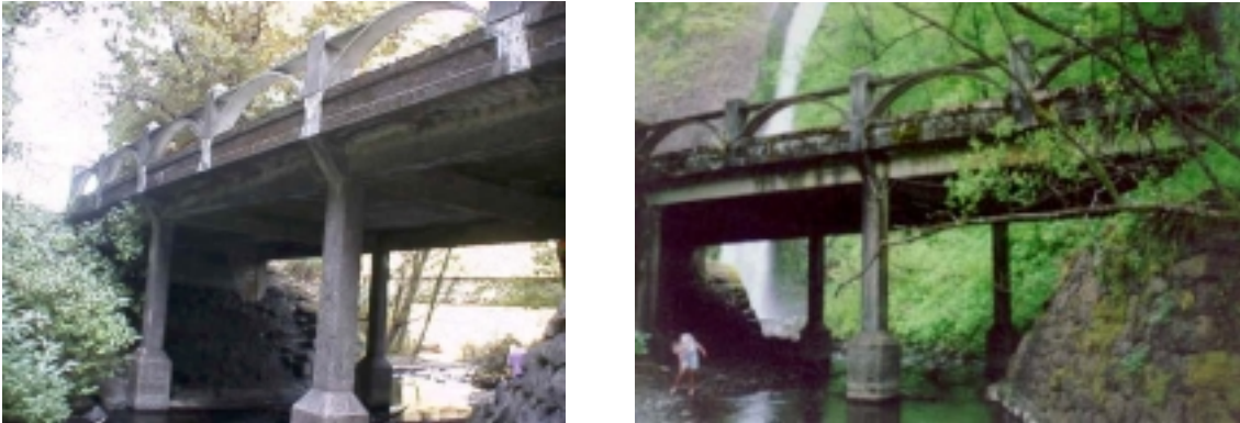
Figure 1.1: Horsetail Creek Bridge (1998, prior to retrofit)
