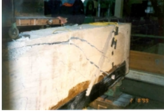
Figure C-35: Diagonal tension crack responsible for failure of F-Only Beam
