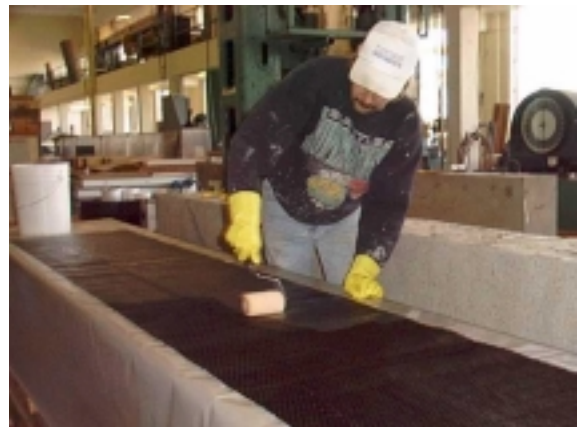
Figure A-11: Saturation of CFRP w/ epoxy
