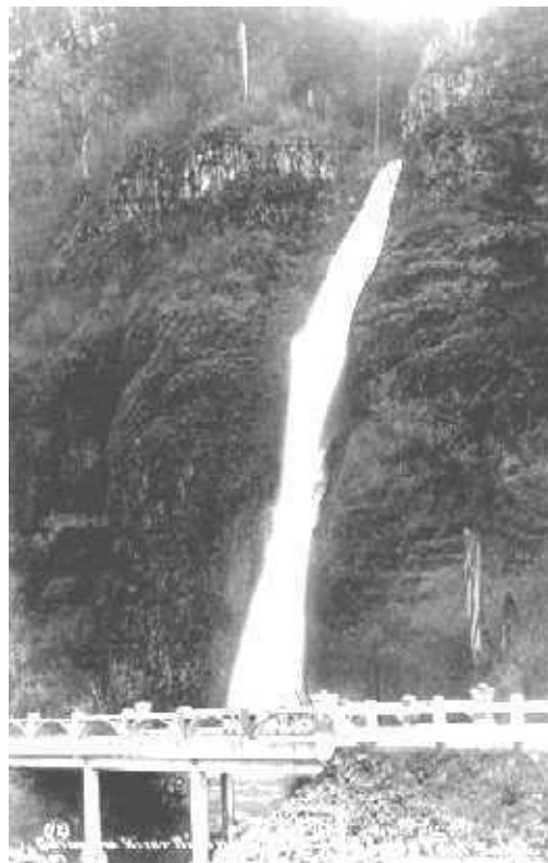
Figure A-2: Horsetail Creek Bridge
