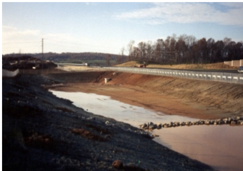
Figure 15. Bioretention Pond 10P-2 as of 10/97
