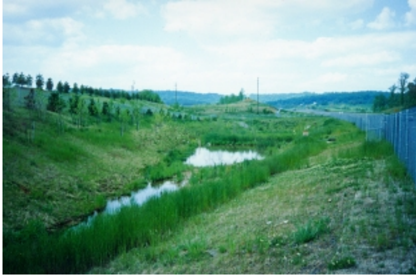
Figure 16. Bioretention Pond 10P-2 as of 05/08/99
