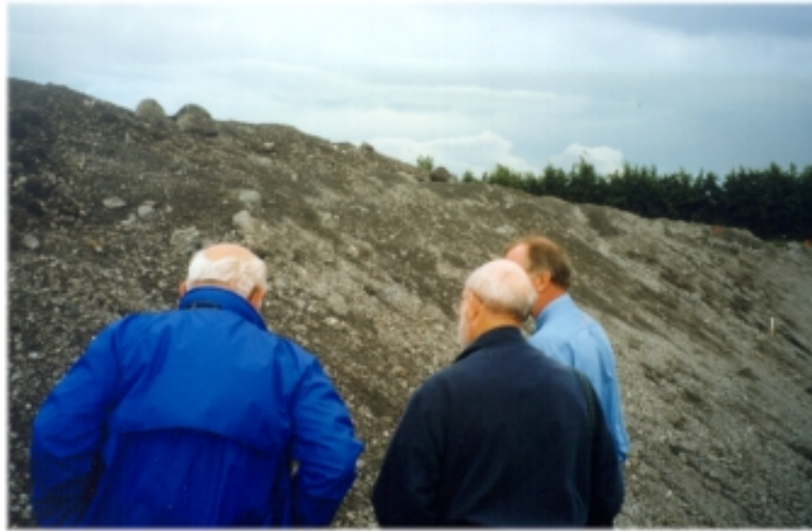
Figure 20. WTE bottom ash use in a road embankment in the Netherlands. The embankment will be about 3 meters high.
