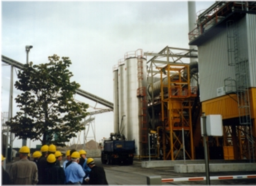
Figure 21. The Swiss-designed Ammann double drum hot recycling asphalt plant in the Netherlands. The plant is co-owned by Vermeer. The plant uses high quantities of RAP that is added to the lower drum. The exhaust gas from the RAP drum is used as burner air for the virgin aggregate drum.
