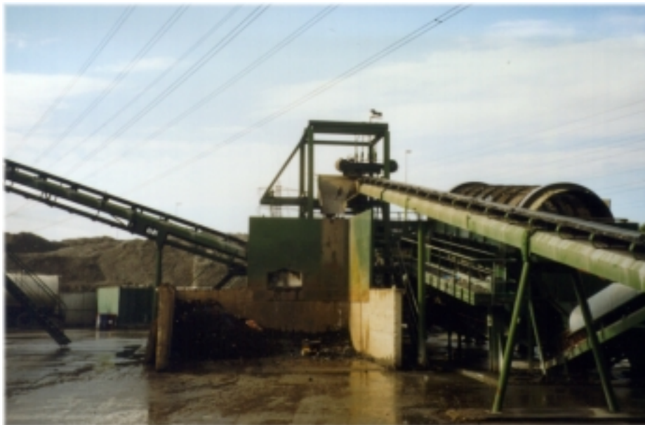
Figure 26. The WTE bottom ash crushing and sieving process at the Jean LeFebvre MSW bottom ash recycling plant in France.
