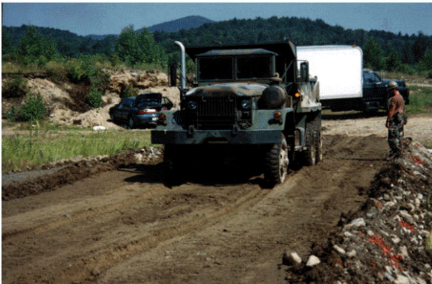
Figure 23. Trafficking the section with a 5-ton dump truck.
