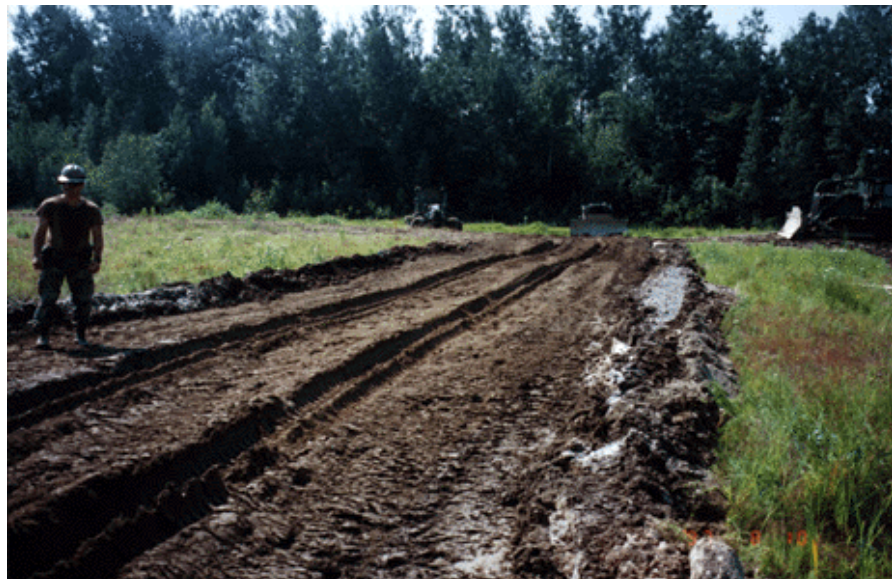
Figure 24. Test section after one pass with a 5-ton dump truck.
