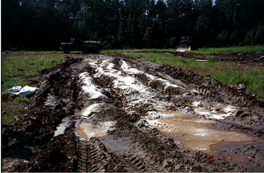
Figure 20. Absorbent spread on test section.
