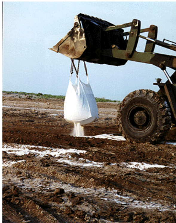
Figure 8. Bucket loader spreading lime.
