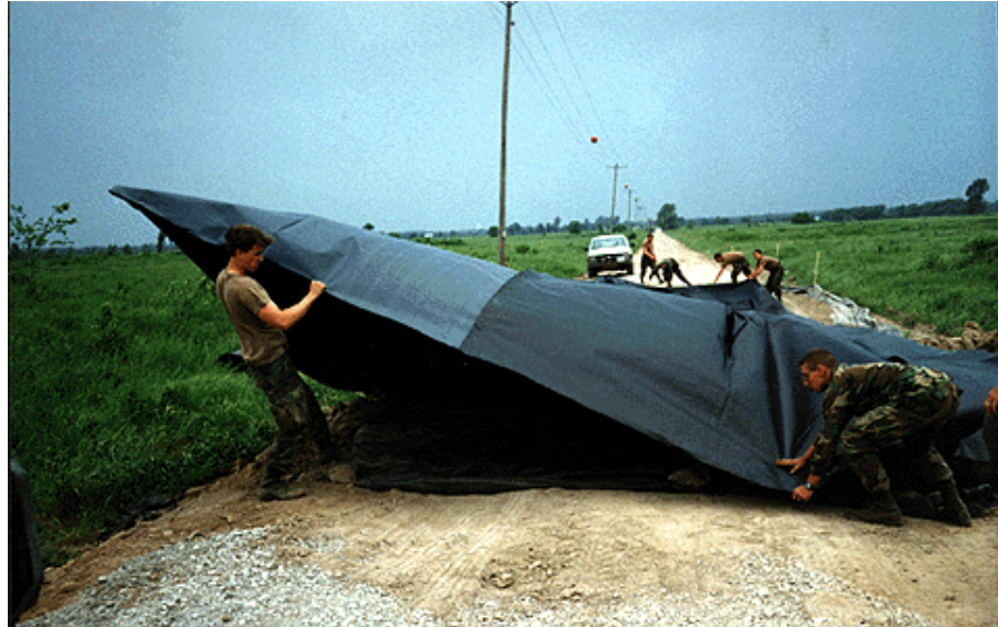
Figure 26. Placing top membrane during light winds.
