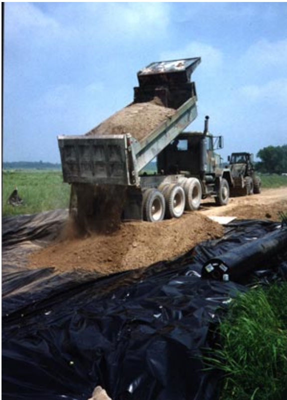
Figure 4. Placing fill soil inside the MESL.
