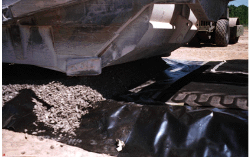
Figure 12. Pan placing gravel on the test section.
