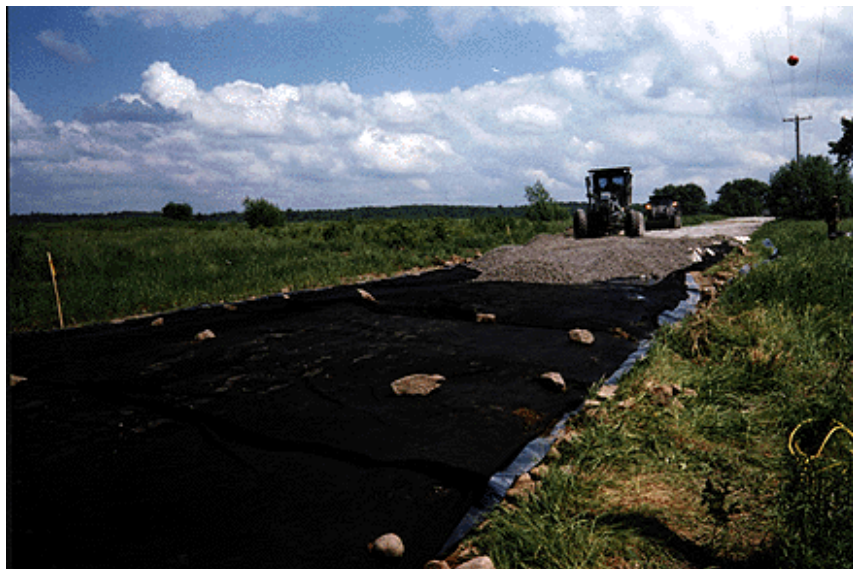
Figure 7. Spreading the gravel wearing course on the MESL.
