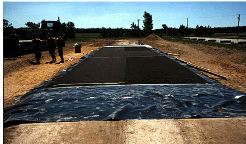
Figure 11. Completed puncture test section before placing a wearing surface.
