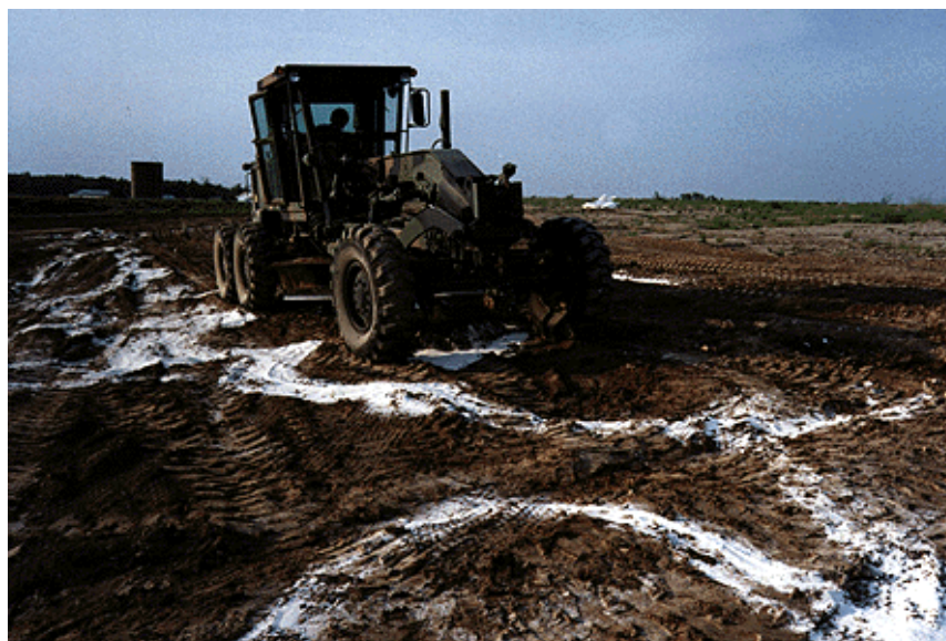
Figure 9. Grader mixing soil and lime.
