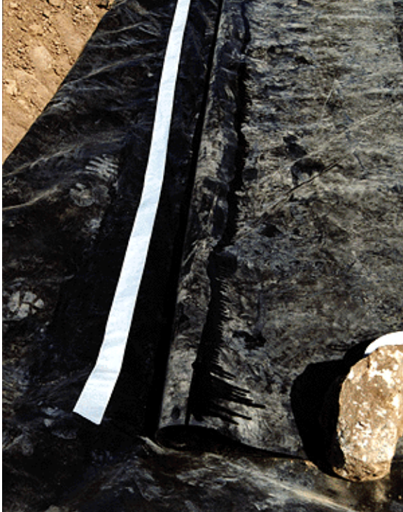
Figure 6. Taping the lower membrane; the upper membrane is being cleaned.
