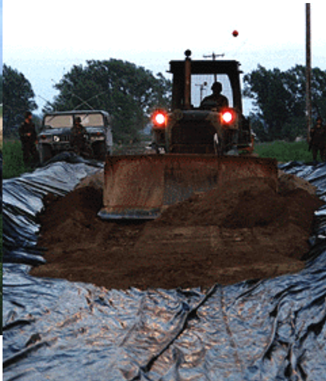
Figure 4. Placing fill soil inside the MESL.
