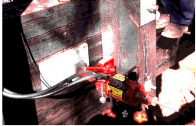
Figure 7—Bar tensioning using a single hydraulic pump and jack.
