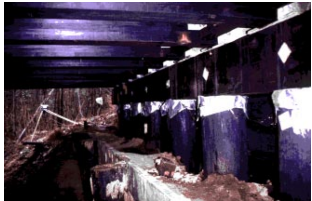
Figure 8—Bridge attachment to the sawn lumber substructure with steel angle saddles.
