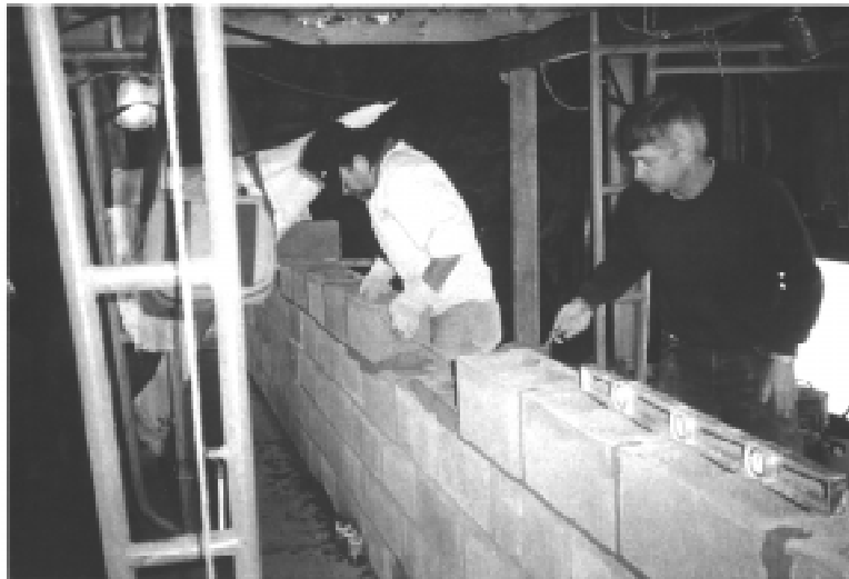
Figure 20. Building the wall.
