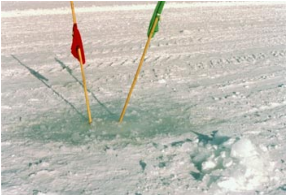
Figure 61. Freshly patched failure site approximately 4 hours after flooding with water.
