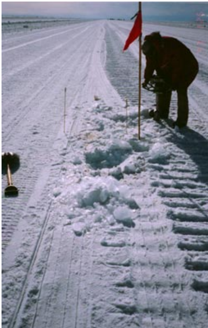
Figure 51. Site of failed runway ice caused by proof cart.
