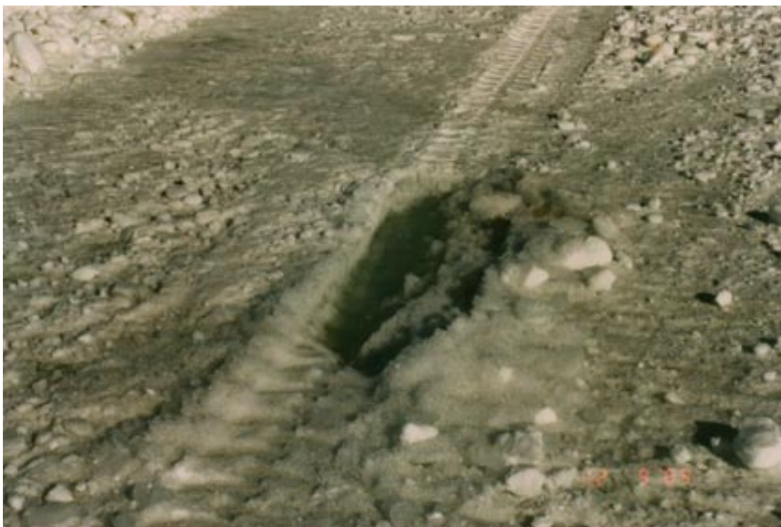
Figure 23. Grader tracks showing breakthrough of thin ice cover over subsurface melt pool.
