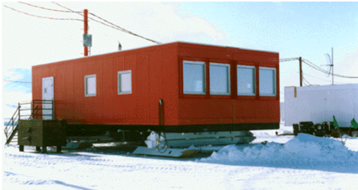
Figure 83. Passenger terminal used during air operations at the Pegasus runway (shown in position at the annual sea ice runway).
