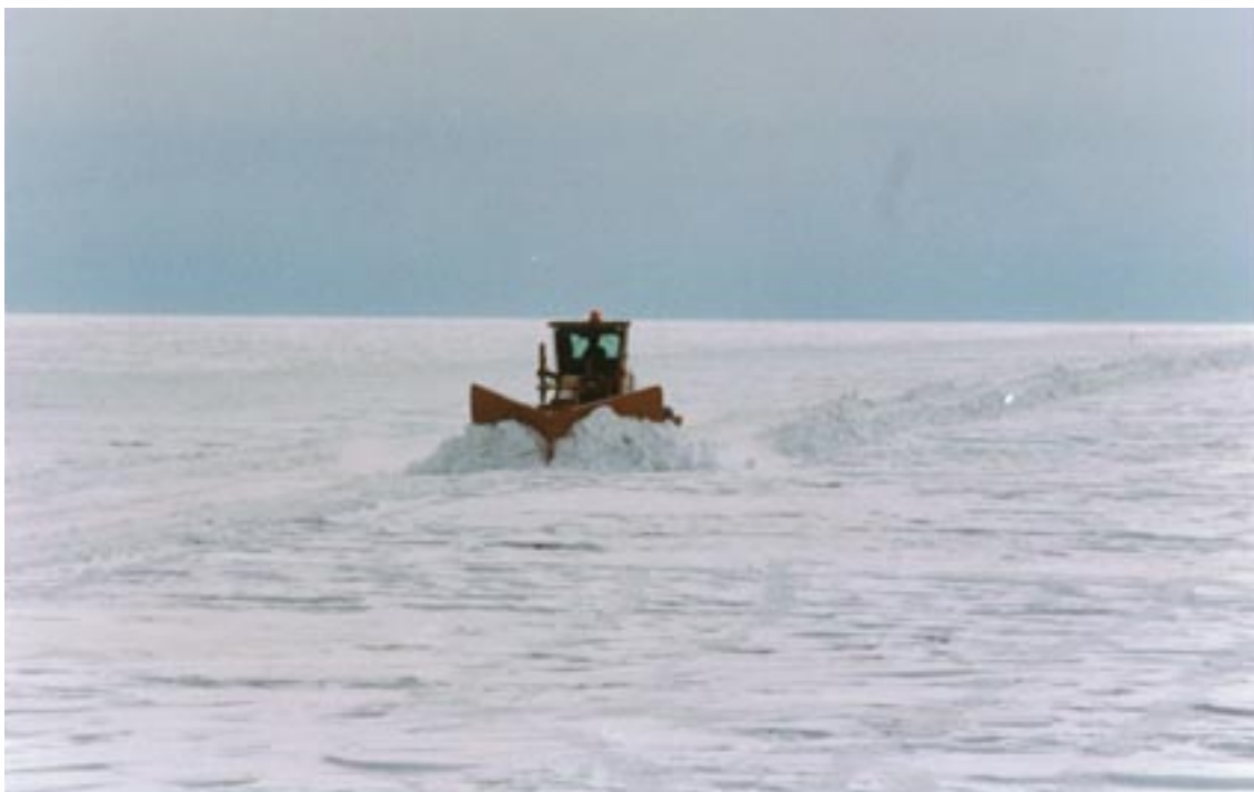
Figure 27. Initial snow stripping on the Pegasus runway using a grader-mounted V-plow.
