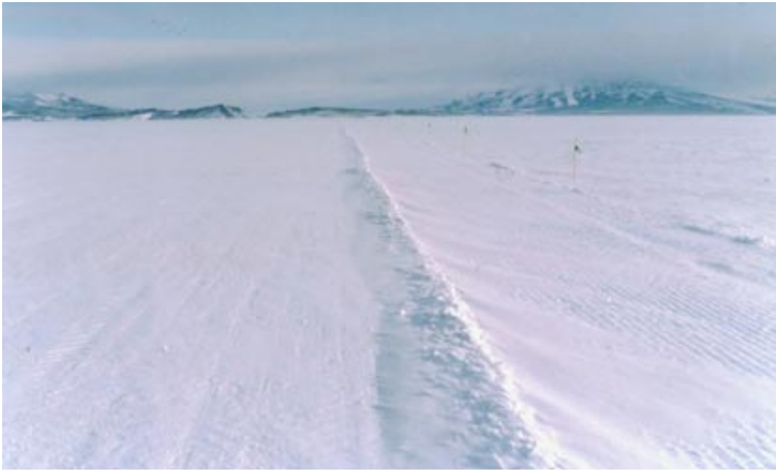
Figure 48. Small windrows trapping blowing snow.
