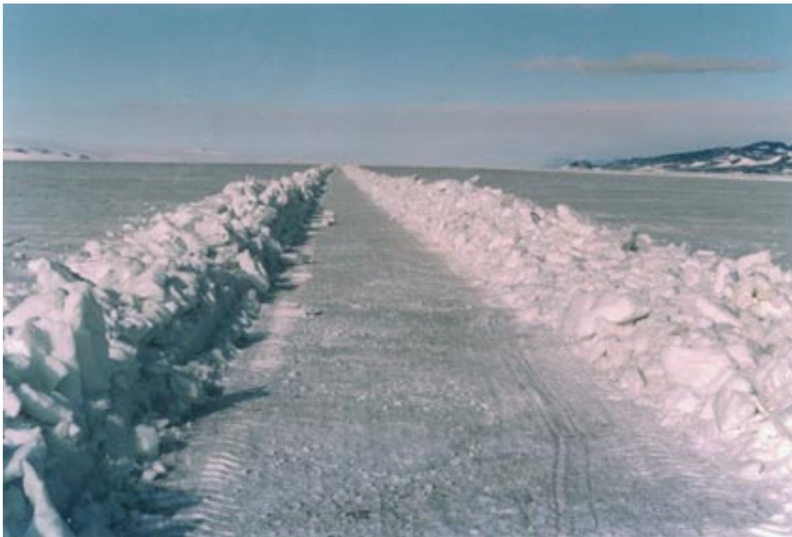
Figure 32. Ice surface following initial snow stripping.
