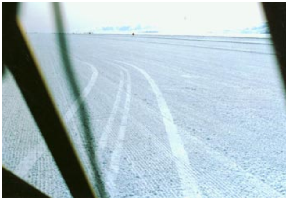
Figure 66. First tracks of aircraft tires on newly constructed glacial ice runway.
