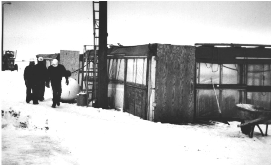
Figure 2. Temporary heated shelter.
