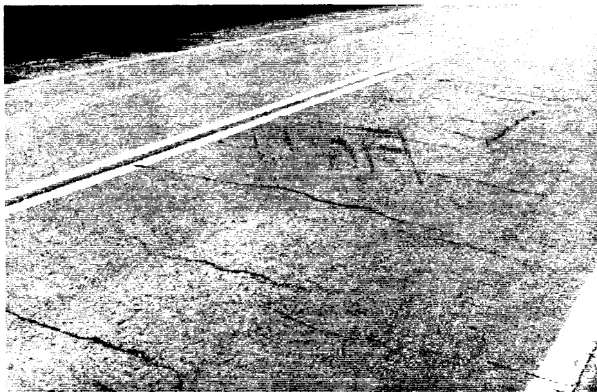
FIGURE 5. Asphalt T-5 (foreground lane) and Asphalt T-6 (background lane)
