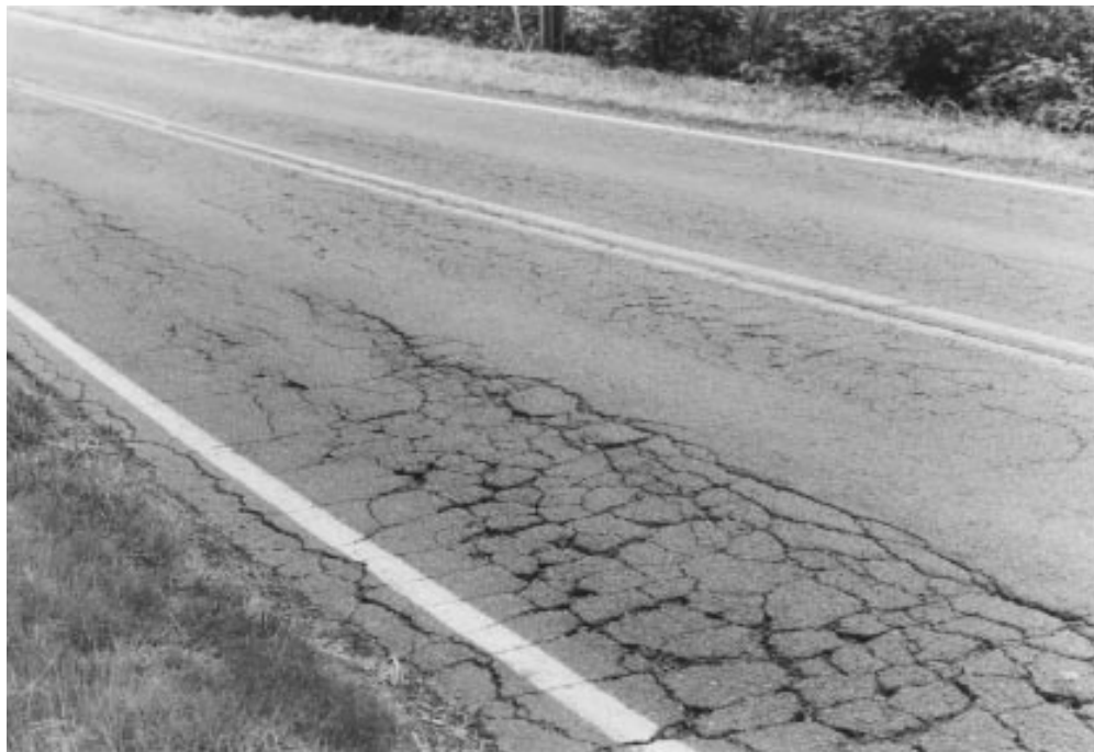
Alligator cracking is a common pavement distress noted during a pavement condition evaluation.
