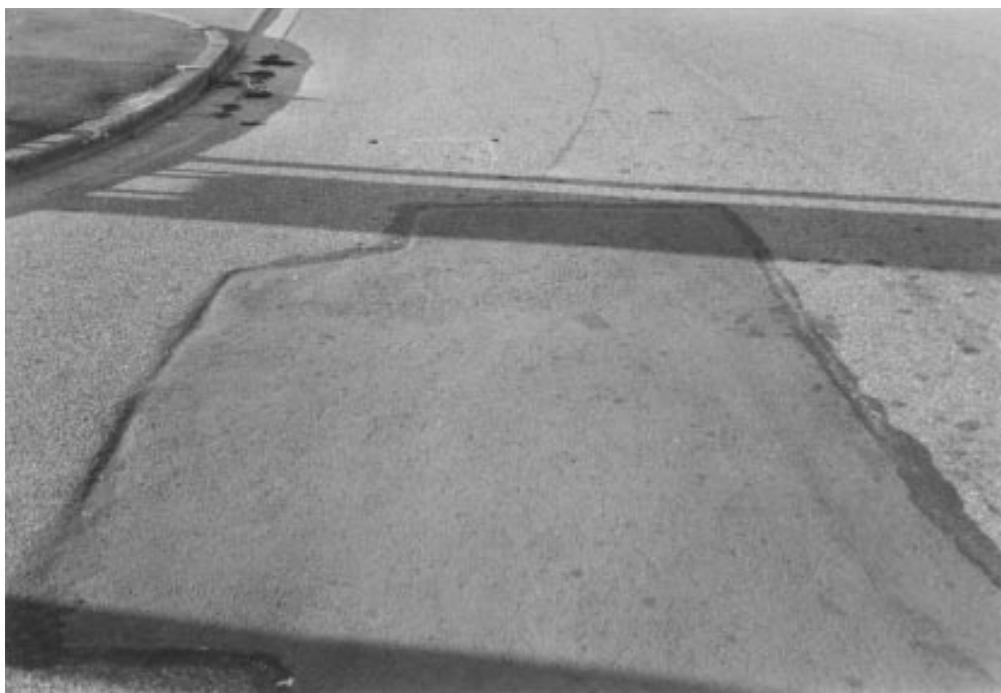
Patching is another commonly used pavement maintenance or rehabilitation activity.
