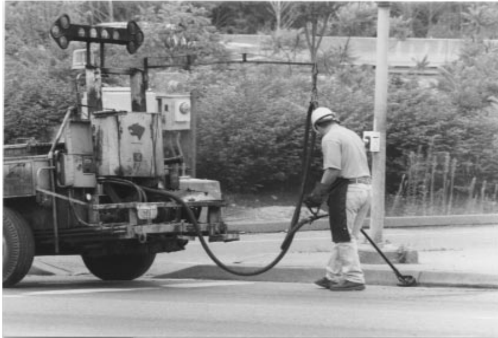
The crack sealing being done on this roadway could be for rehabilitation or maintenance purposes.
