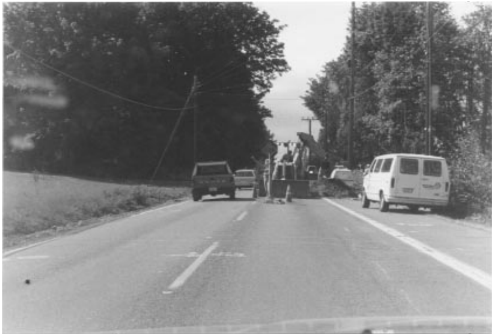
A backhoe is used for a test pit to get information about the material underlying the roadway.
