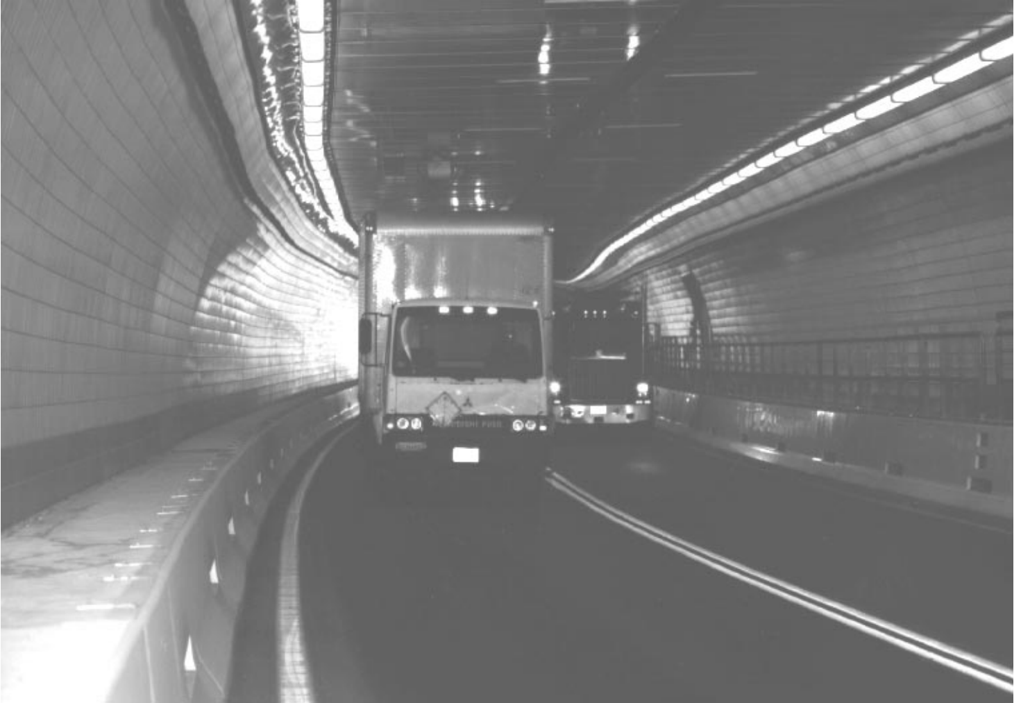
Figure 2: The Ted Williams Tunnel
