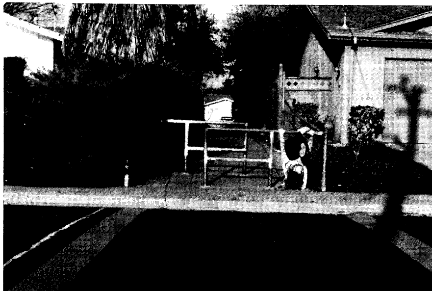
Midblock crosswalk and barrier at end of midblock pedestrian passageway.
