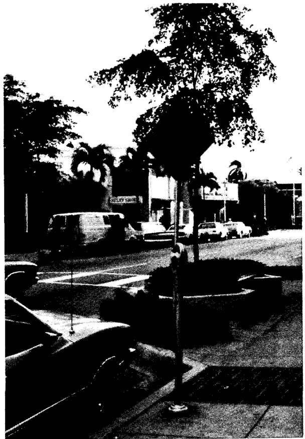
Midblock crosswalk; sidewalks extended into parking lane giving greater visibility of pedestrians and shorter walking distance.
