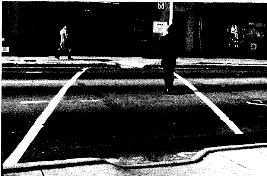
Curb-cut ramps for elderly and wheelchaired pedestrians.
