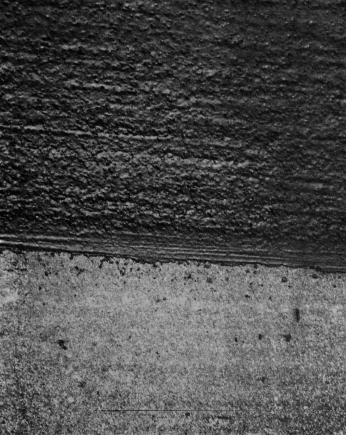
FIGURE 2-2. AGGREGATE SLURRY SEAL
