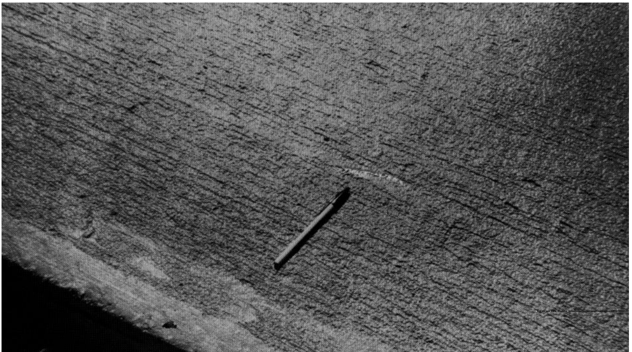
FIGURE 2-4. HEAVY BURLAP DRAG FINISH
