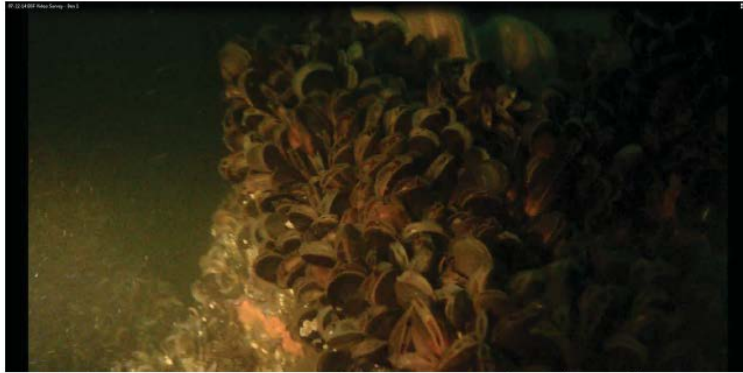
Figure 16. Blue mussels on steel pile of the TidGen mooring structures (ORPC Maine LCC 2015).
