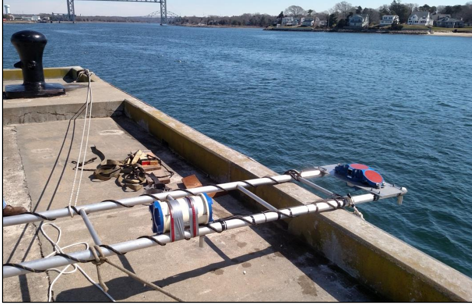
Figure A-8: Photograph looking eastward at the corner of the MMA pier, showing the H-ADCP (far right) mounted at the bottom of the mounting structure. The white canister (blue caps) is the external battery housing used to power the H-ADCP. The canister top was a distance 1.98m above the H-ADCP. The H-ADCP was installed at an elevation approximately -1.05m below the MLLW tidal datum.
