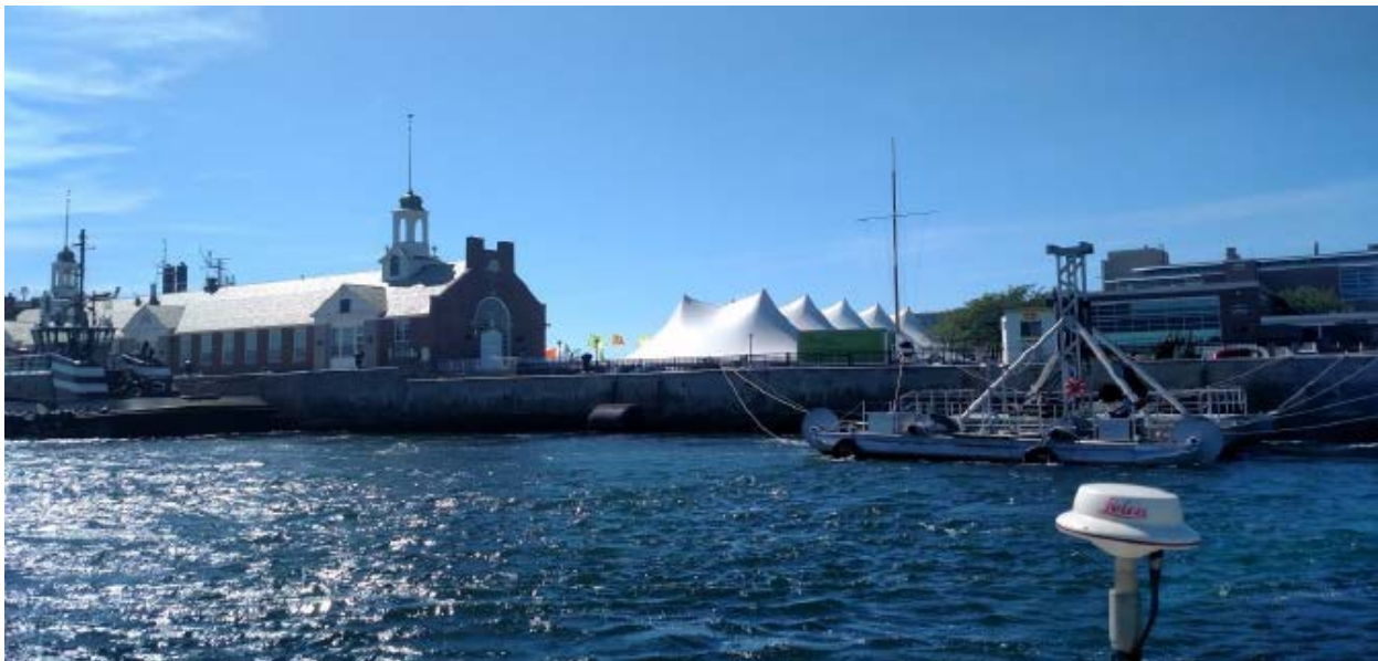
Figure 29. The MMA pier and Joule test device on August 5, the day of the survey. Note the tugboat docked along the pier to the left of the photo, about 35-40 meters downstream of the pontoon barge (for scale, the pontoon barge is 35 feet in length). In the foreground is the GPS antenna.
