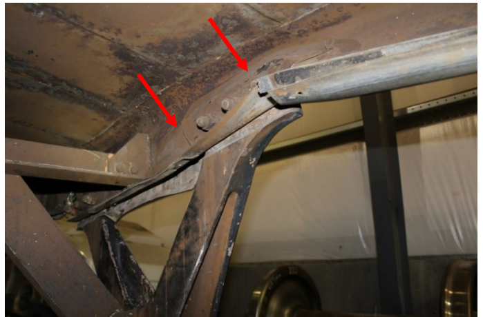
Figure 17. M1 side sill front left truck connection (interior view)
