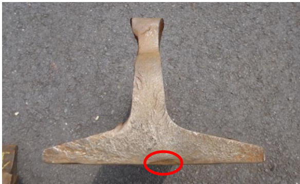
Figure 7. Rail Base Defect at New York
