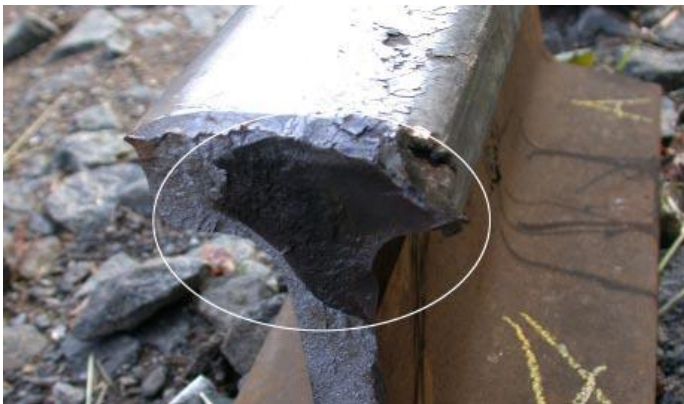
Figure 3. Broken rail and rail surface damage at New Brighton (12)
