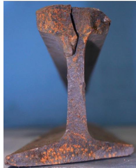
Figure 6. Vertical Split Head from the rail at Mount Carbon, WV
