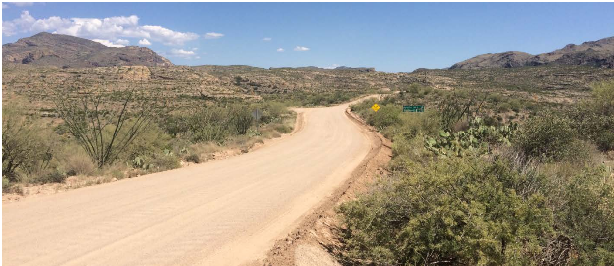
Figure 8: A relatively flat stretch of the Apache Trail on the unpaved section.
