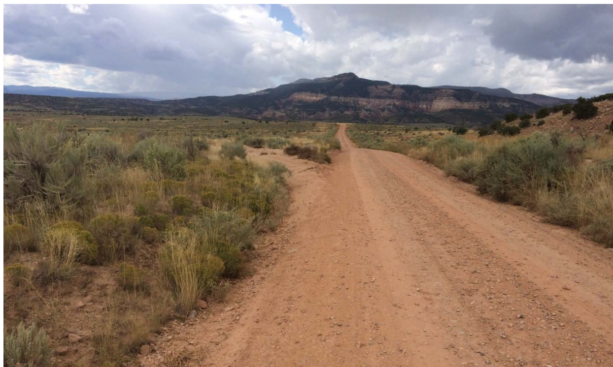
Figure 1: Relatively straight section of FR 151 between the road's start at U.S. Route 84 and the Rio Chama.
