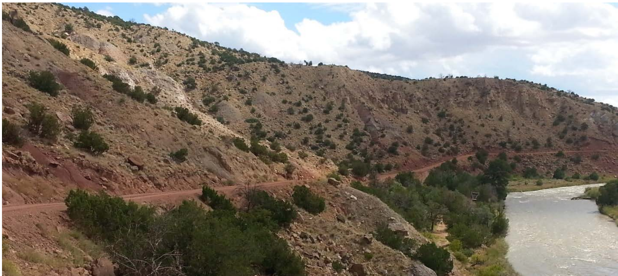
Figure 6: FR 151 adjacent to the cliffs near Mile Post 6
