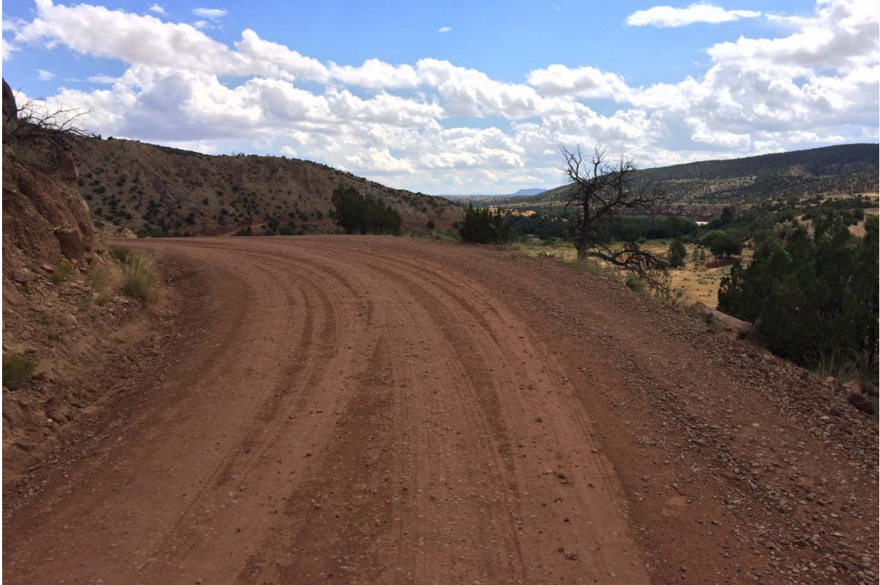
Figure 7: Limited sight distance curve near Mile Post 6
