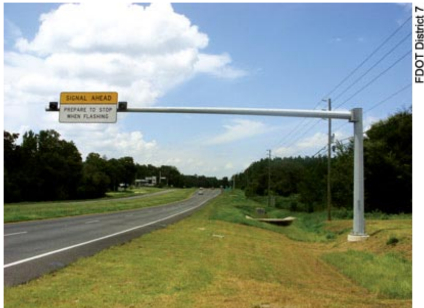
These before (top) and after (bottom) views show installed overhead signage, another example of a safety improvement on a local road in District 7.
