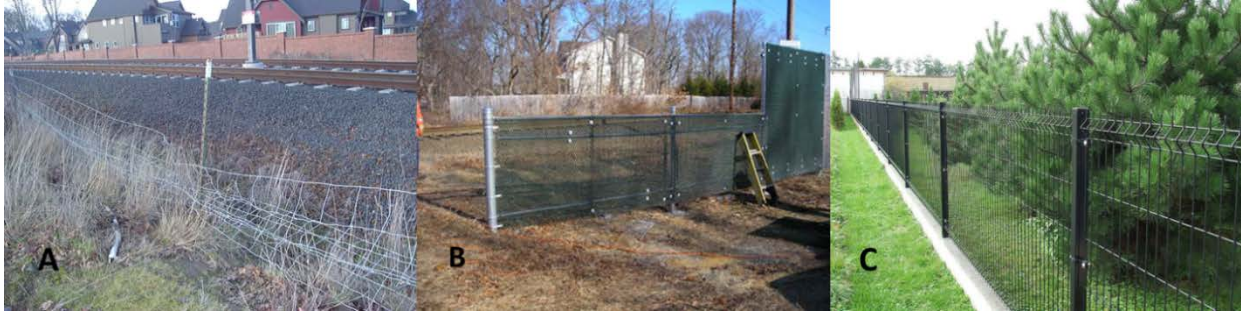
Figure 9. Examples of Fencing Along Railroad Rights-of-Way
