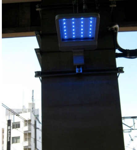
Figure 3. Blue LED Lights in Japan Railroad Station Platforms 18
