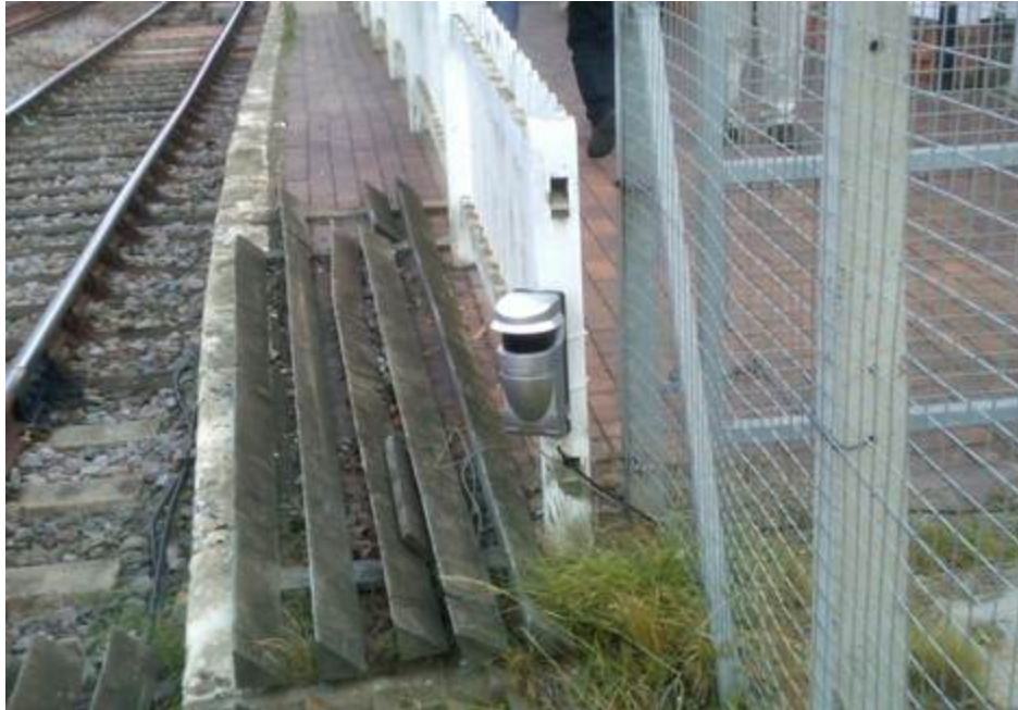
Figure 14. Track Surveillance with Laser Beam in UK 52
