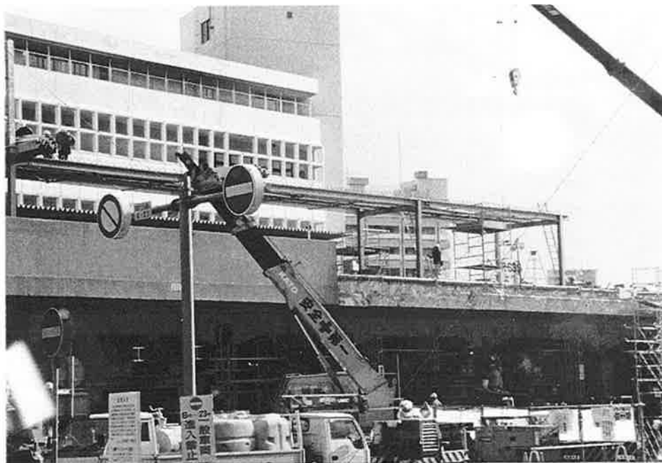
JRT-45. Rokkomichi Station replacement.
