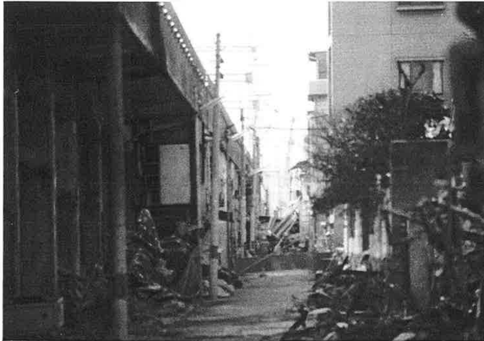
HER-33. This barrier is visible in following photograph. There is minimal damage to the viaduct but residential damage prevents our access. This is the western limit of the viaduct damage.
