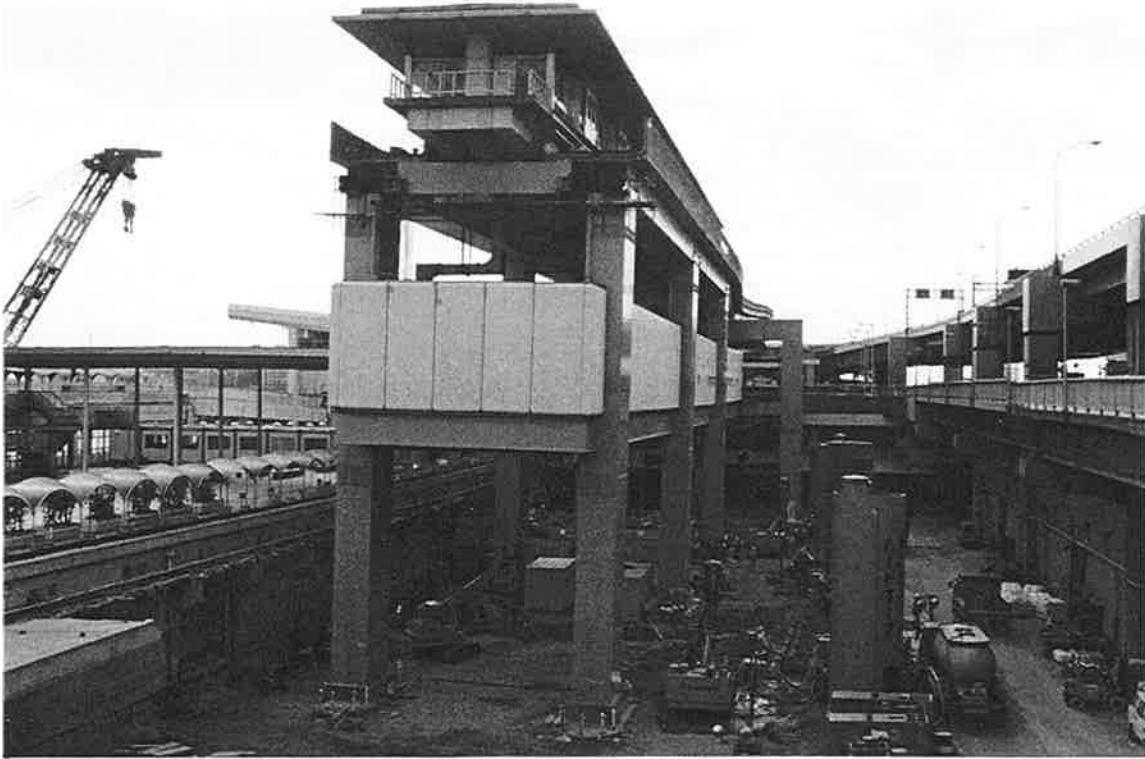
PI-9. A close-up of the tower shows it is the Port Island Station.
