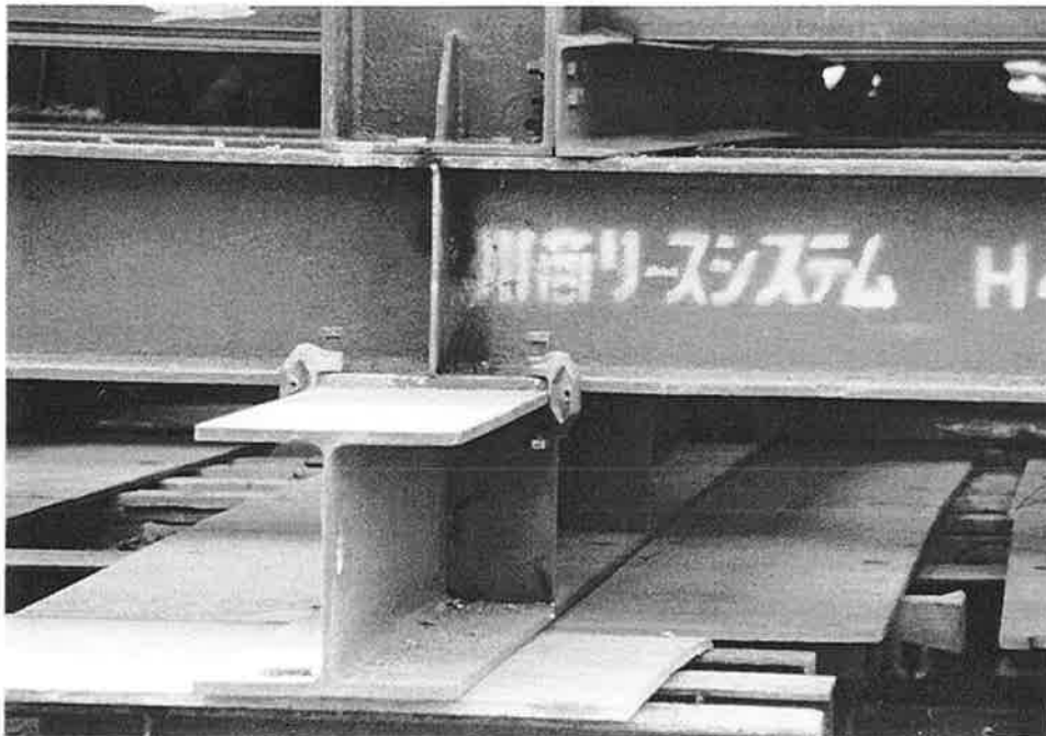
JRT-22. Lateral restraint on this temporary support appears by C-clamp.
