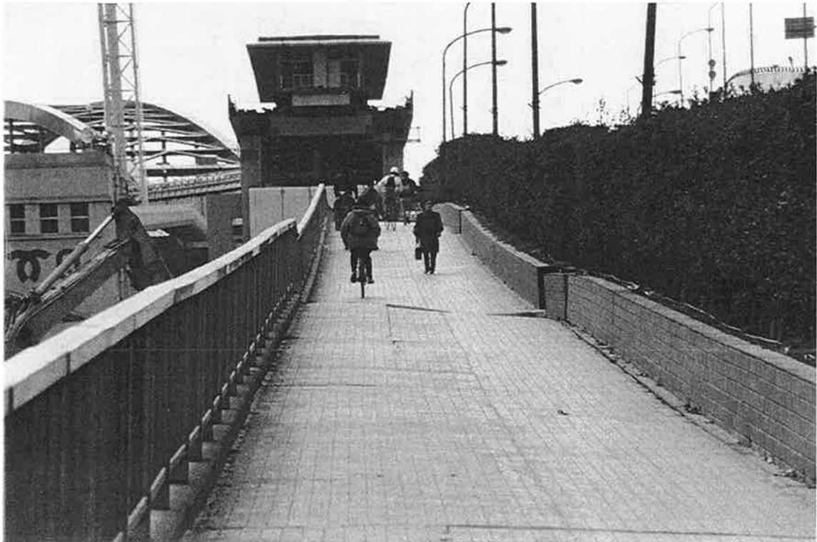
PI-10. The pedestrian bridge approaches the Port Island Peoplemover Terminal Station that is integral with the marine terminal. Note the slope and settlement.
