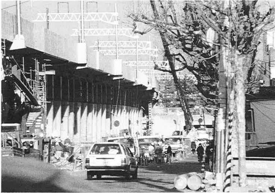
JRT-37. Steel jacket repairs at the tops of the columns.
