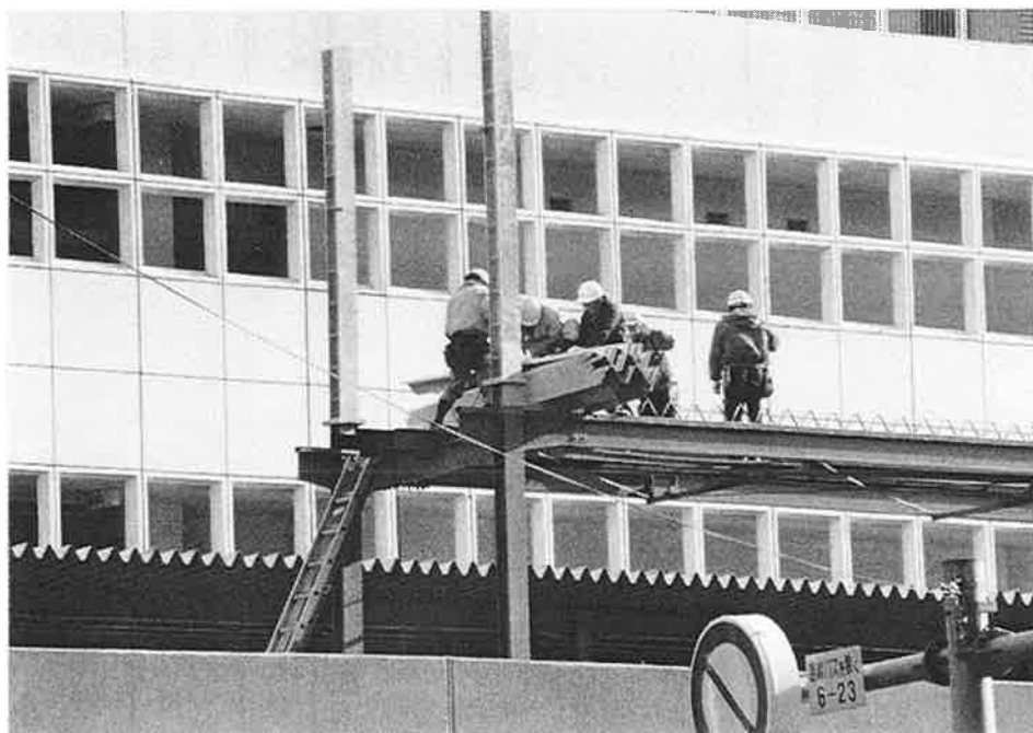
JRT-46. Construction of the new platform for Rokkomichi Station.
