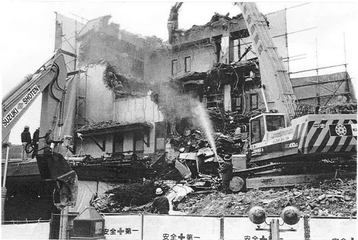
HC-11. Shukugawa Station demolition
