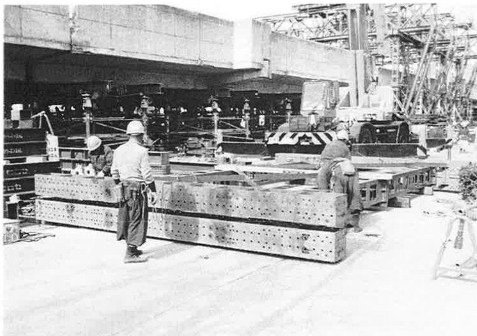
JRT-10. Construction of additional jacking frames.
