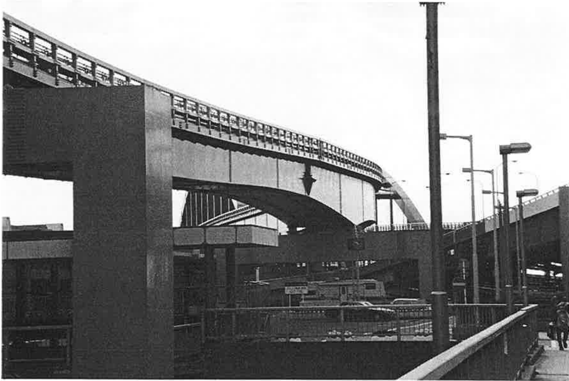
PI-11. The steel box girder span approaching the arch span was undamaged.
