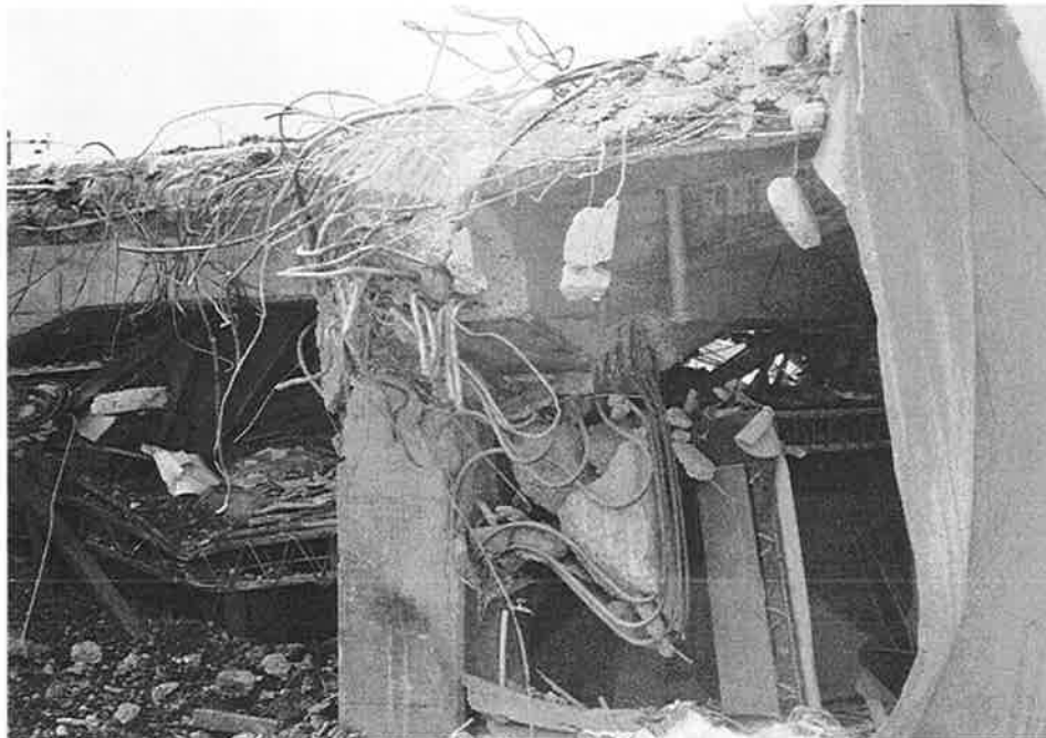
HER-10. Beginning of the failed viaduct; the steel members were used for residential and commercial buildings constructed under the viaduct.
