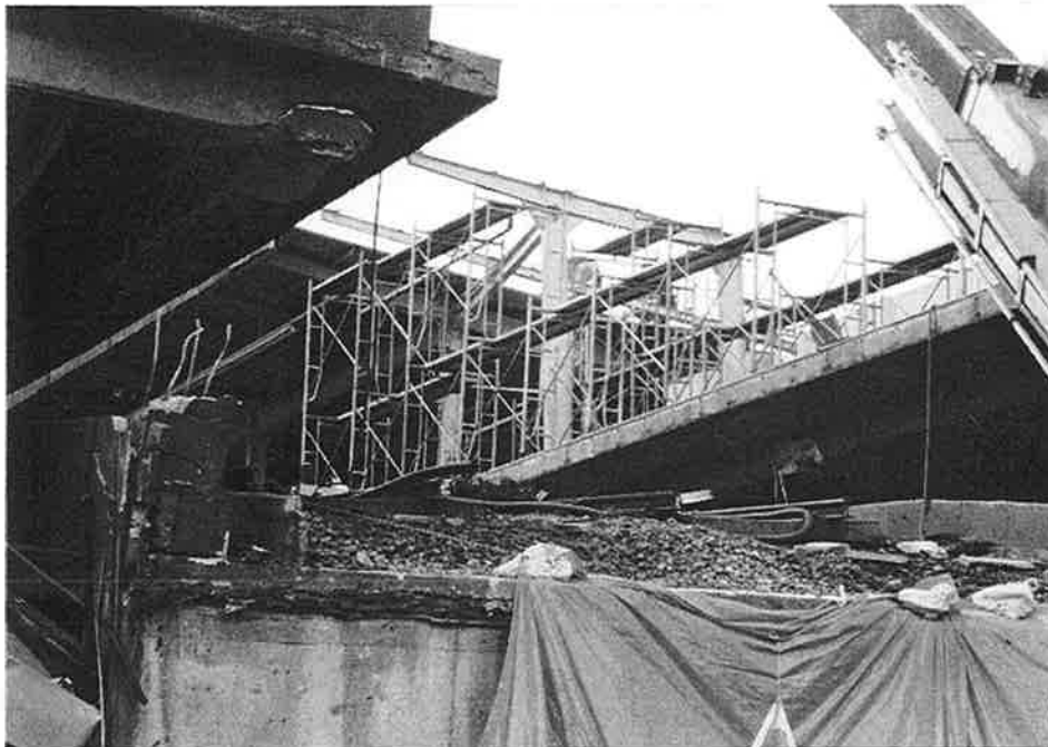
HER-28. Demolition is underway at Shinzaike Station.
