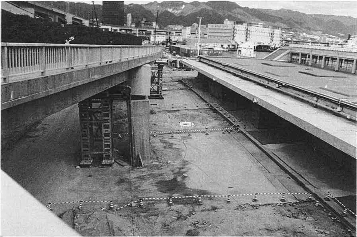
PI-5. The foundations like the bolt circle in the center are all that remain of the Port Island peplemover. A pedestrian bridge is to the left. Downtown Kobe is in the background.
