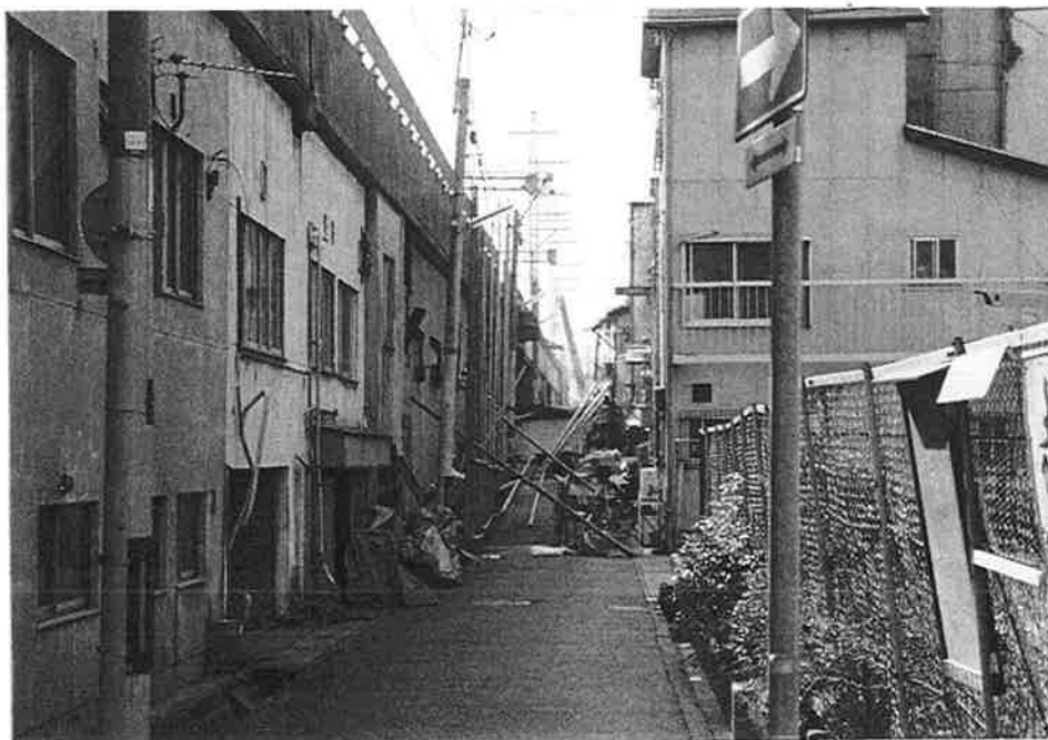
HER-36. The viaduct to the left is undamaged, but our progress is stopped by the damage to lighter construction.
