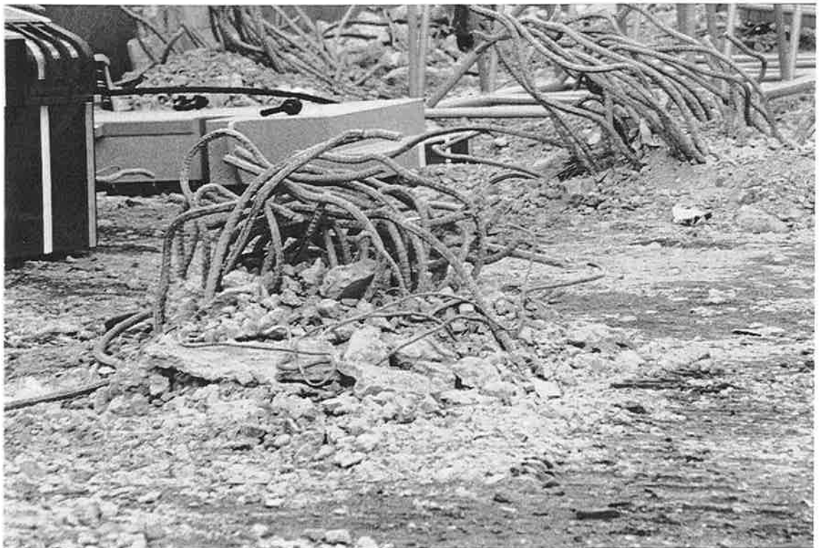
HC-17. Remnants of the failed viaduct
