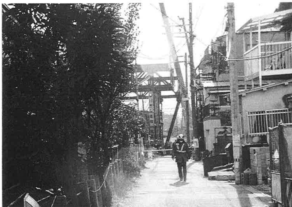
JRT-47. Housing adjacent to the viaduct was damaged but still standing. The viaduct partially collapsed in this area. Note the jacking frames in the background.
