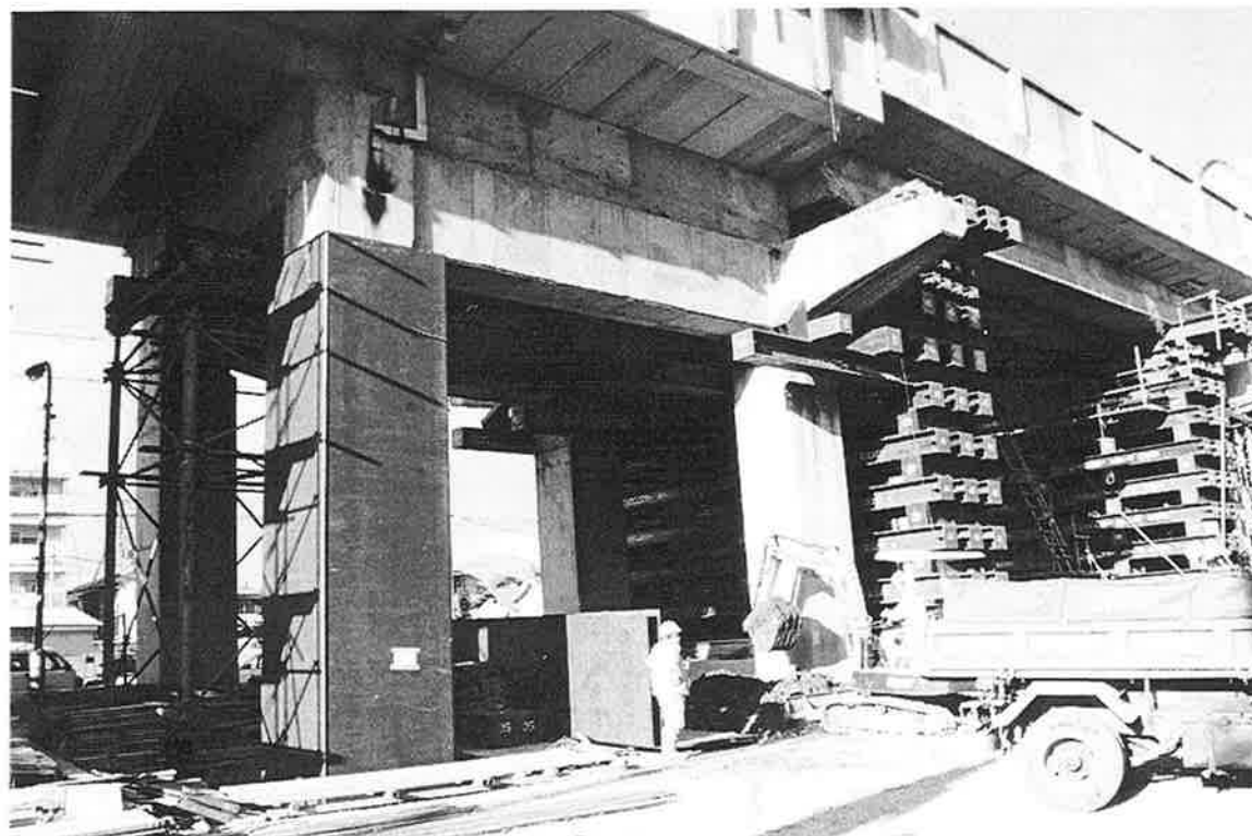
JRS-20. The drop in span on the right was lifted off the ground and relocated on the piers. The adjacent spans were stiffened with the additional girder. Steel jackets were applied to columns.
