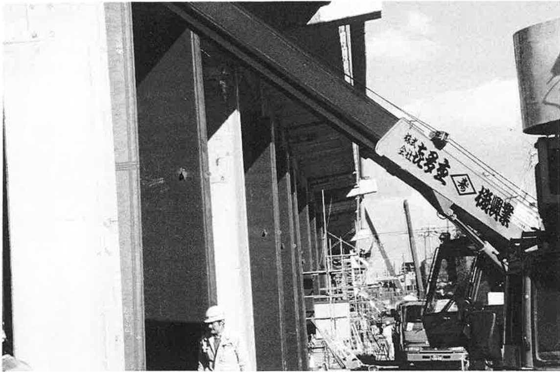
JRS-15. Many steel jackets are installed.
