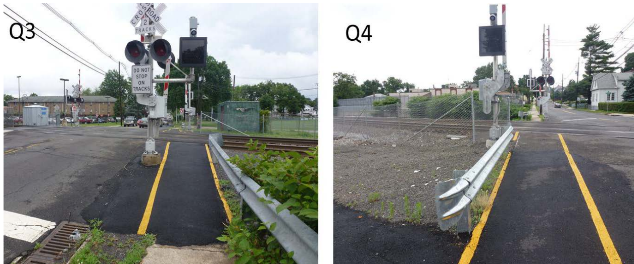
Figure 7. Added Safety Enhancements in Quadrant 3 (left) and Quadrant 4 (right) in August 2012
