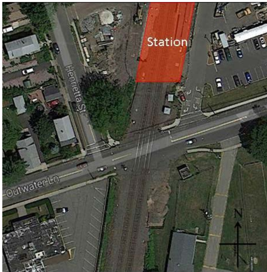
Figure 2. Outwater Lane Grade Crossing in Garfield, NJ
