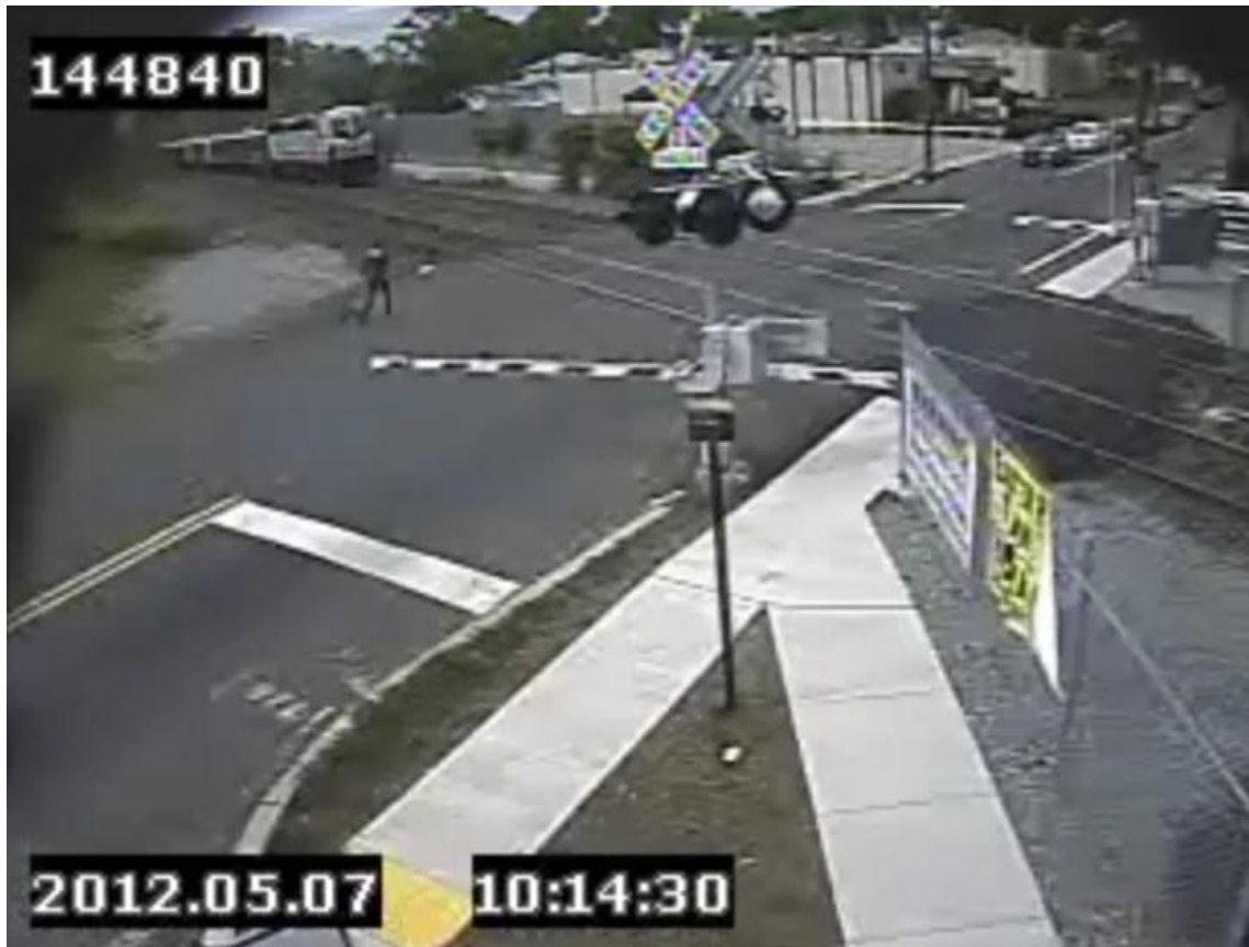
Figure 17. Pedestrian Violation Prior to Second Train Warning System Installation
