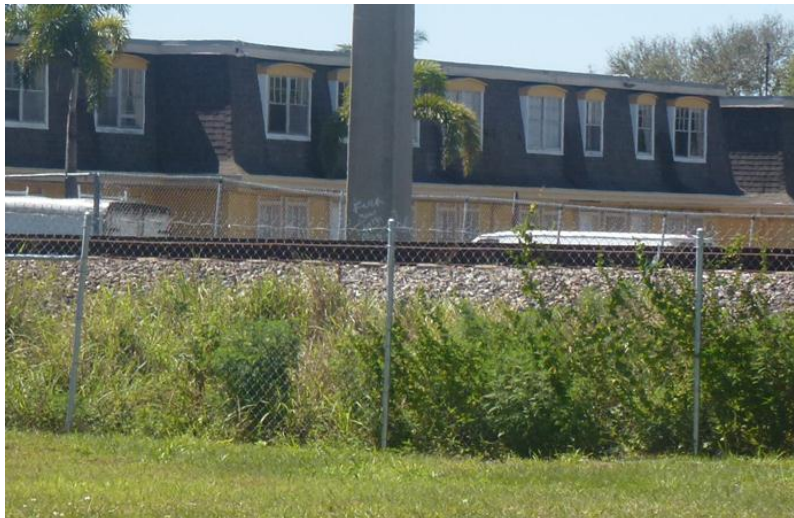
Figure 24. Fence on SFRC ROW between 45 th and 36 th Streets (September 2012)
