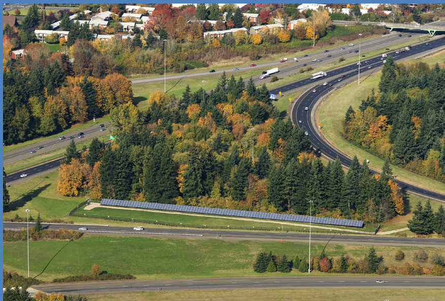
Figure 13: Aerial view of the Oregon Solar Highway. (Courtesy of Oregon DOT)
