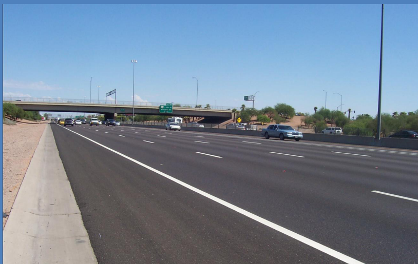
Figure 5: Rubberized Pavement on Interstate 10 near Phoenix, Arizona. (Courtesy of ADOT)
