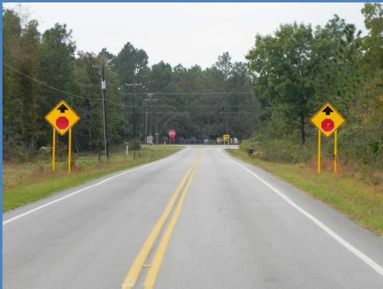
Figure 2: Photo of doubled up (left and right) signing to warn drivers of an upcoming stop sign. (Courtesy of SCDOT)
