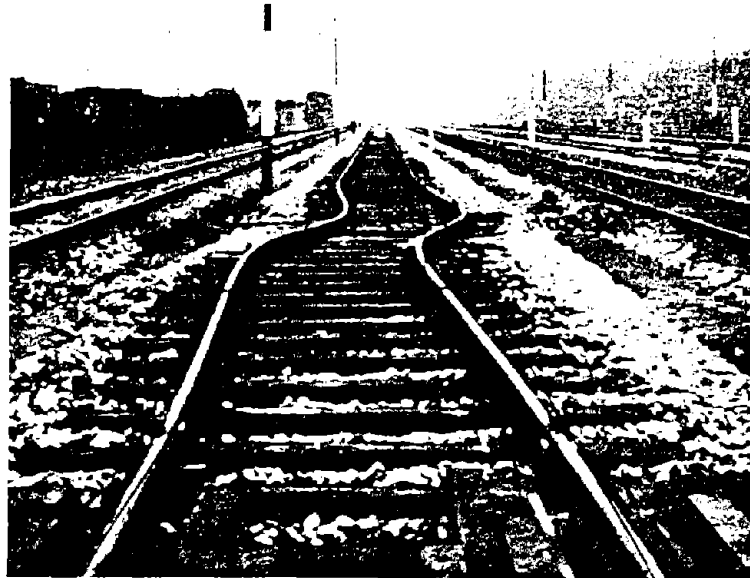
(a) Nearly antisymmetrical buckling mode [7].
