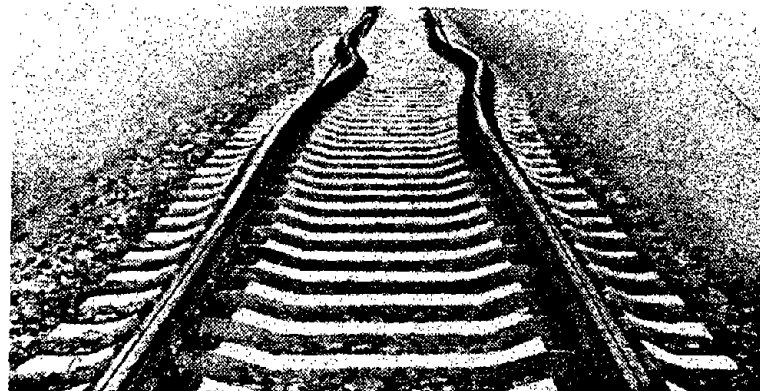
(b) Nearly symmetrical buckling mode [12].
