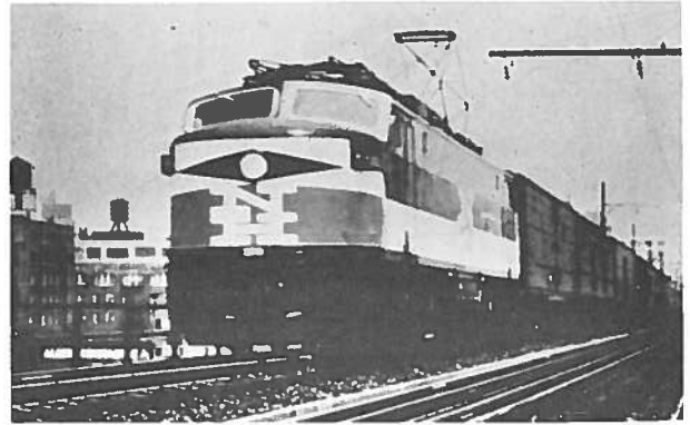
FIGURE 8 NEW HAVEN EP5, IGNITRON RECTIFIER LOCOMOTIVE, 4000 HP, 11 KV, 25 HZ
