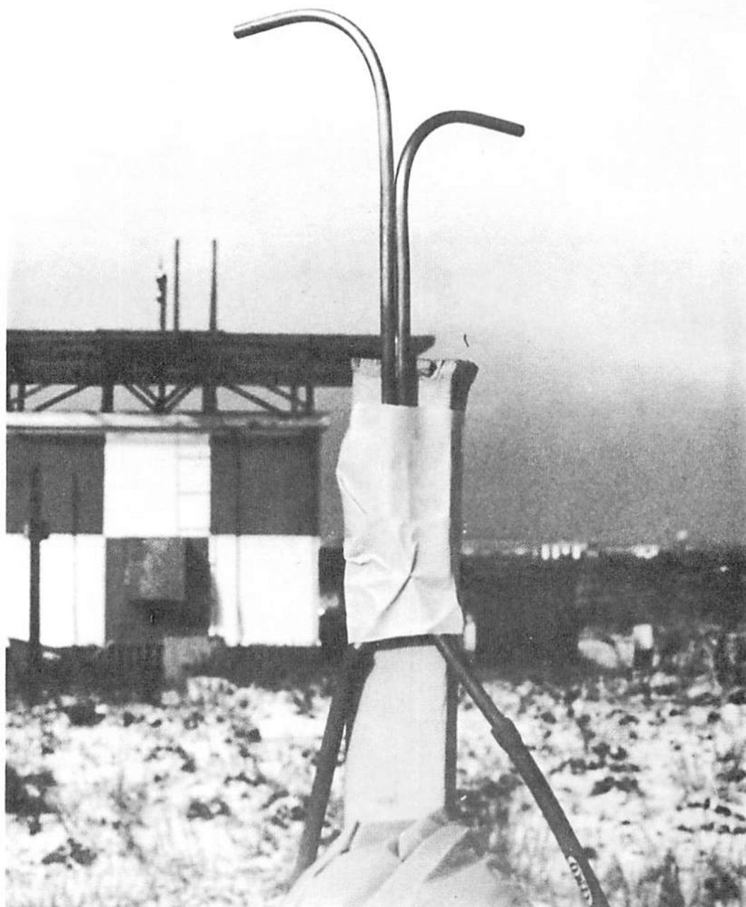
Figure 46. 120° Dual Pitot Tube Installed at Kennedy 31R Middle Marker. (The Tubes are Made of 1/4" Copper Tubing.)
