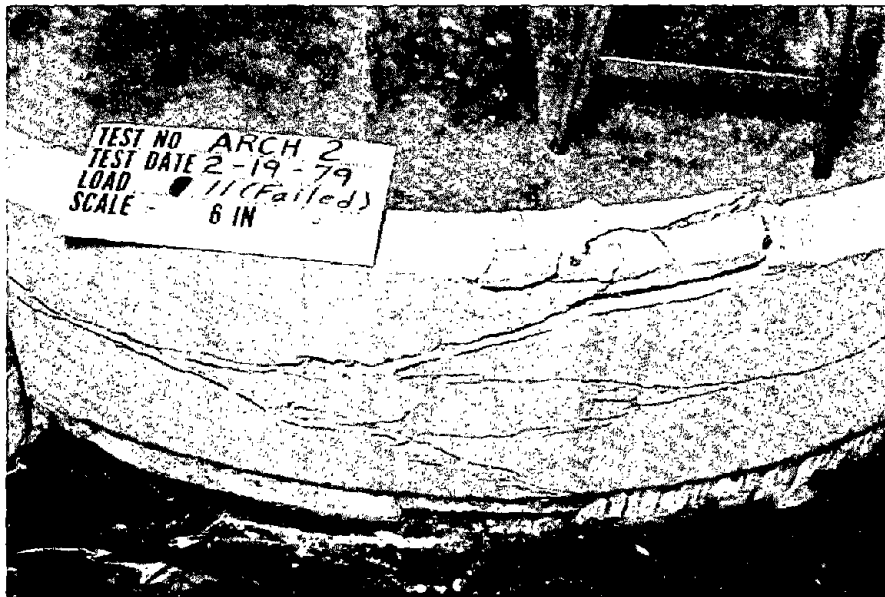
FIGURE 4.64 CROWN OF ARCH-2 AT FAILURE
