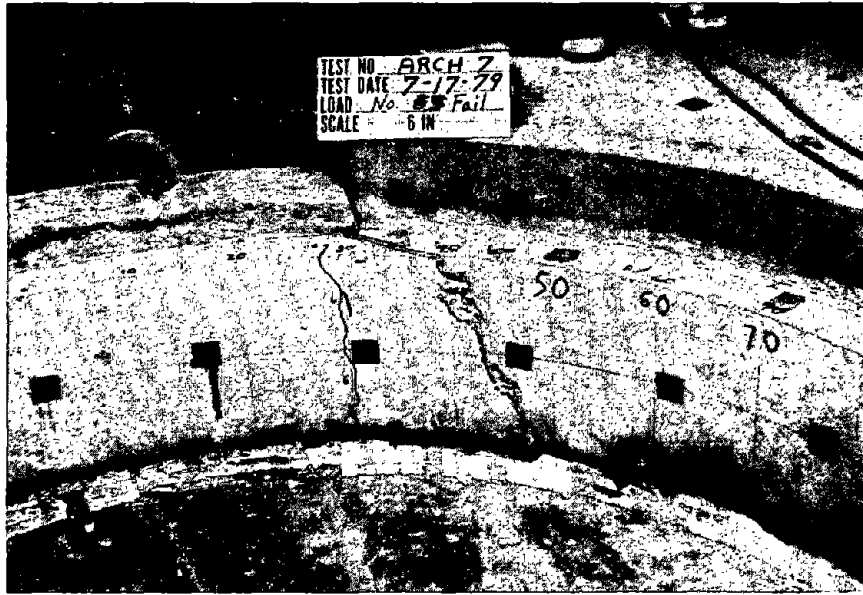
FIGURE 4.75 ARCH-7 AT FAILURE
