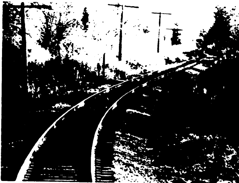
Fig. 3.4 REVERSE CURVE 6^{\circ}20' TO 4^{\circ}54'
