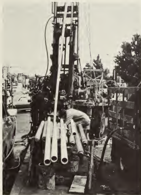
FIGURE 7-7. INSTALLATION OF PVC GEOPHYSICAL/ INSTRUMENTATION CASING
