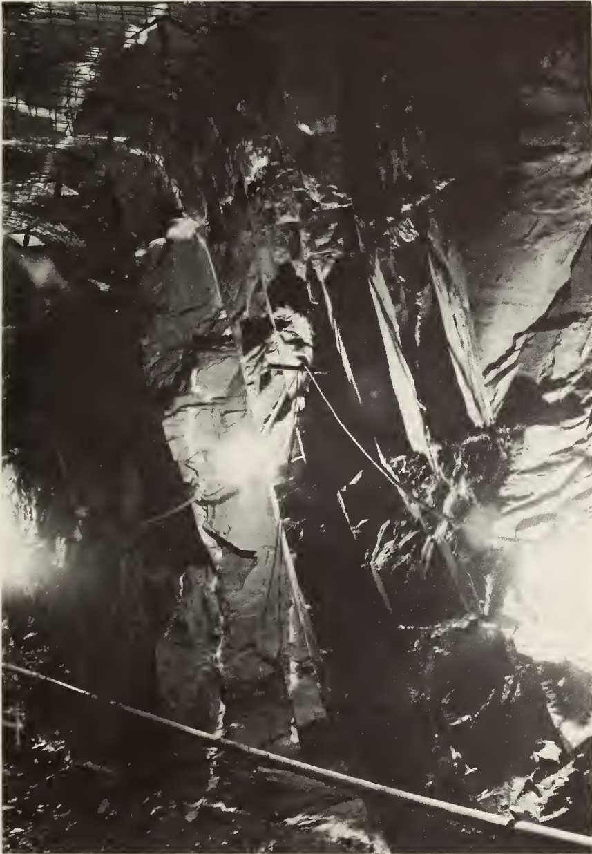
FIGURE 9-4. STRUCTURAL DISCONTINUITIES, PORTER SQUARE PILOT TUNNEL
