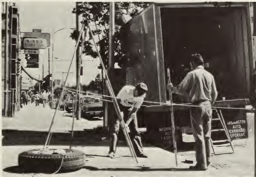
FIGURE 7-51. PREPARING FOR INSTALLATION OF NUCLEAR SONDES IN BOREHOLE
