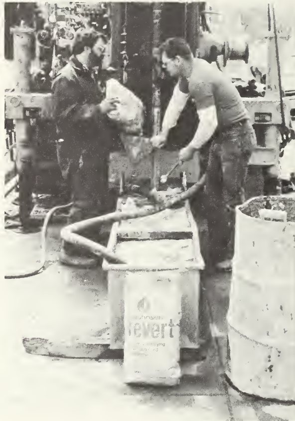
FIGURE 7-3. MIXING REVERT™ DRILLING FLUID ADDITIVE IN THE MUD RESERVOIR
