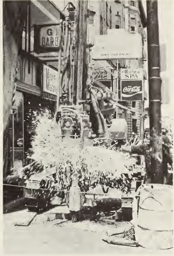
FIGURE 7-17. "UNPLUGGING" THE ODEX BIT
