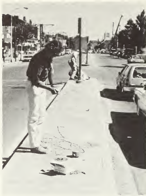
FIGURE 7-60. PREPARING "SHOT HOLE" FOR CROSSHOLE SEISMIC SURVEY
