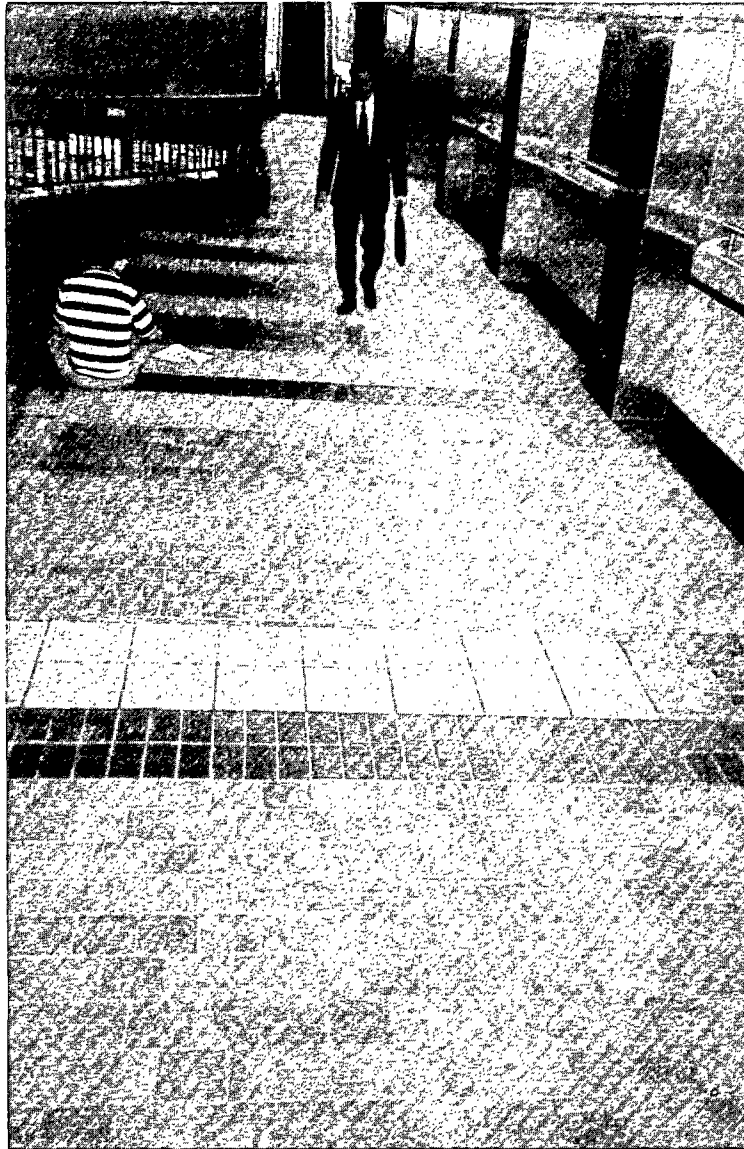
Figure 3-8 Arrangement of Detectable Warning Materials at MBTA South Station Test Site
