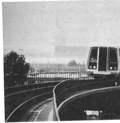
Elevated structure on the Washington
