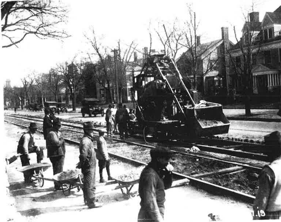
Labor intensive, early track maintenance.
