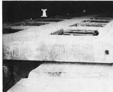
Typical section of floating slab track construction.
