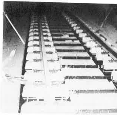
Duo-block concrete ties are increasingly used with slab track to limit vibration.
