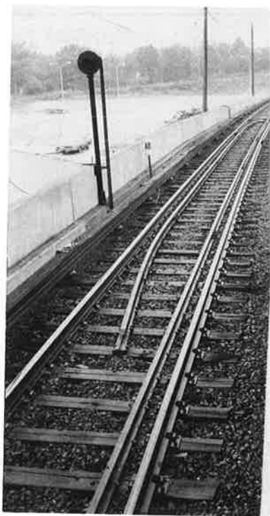
Tie and ballast track with power rails.
